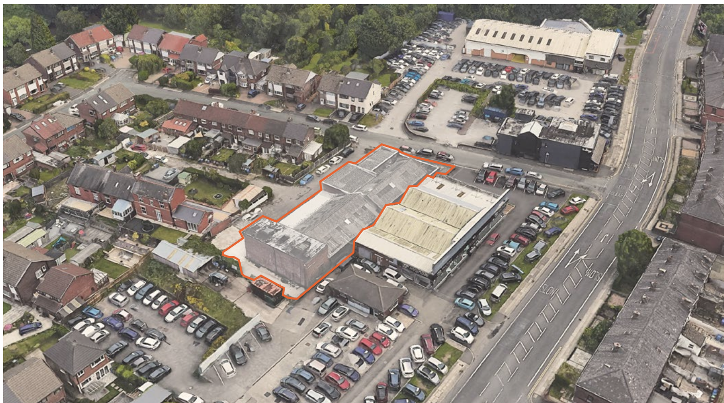
FIGURE 5 | AERIAL VIEW LOOKING SOUTH EAST.
