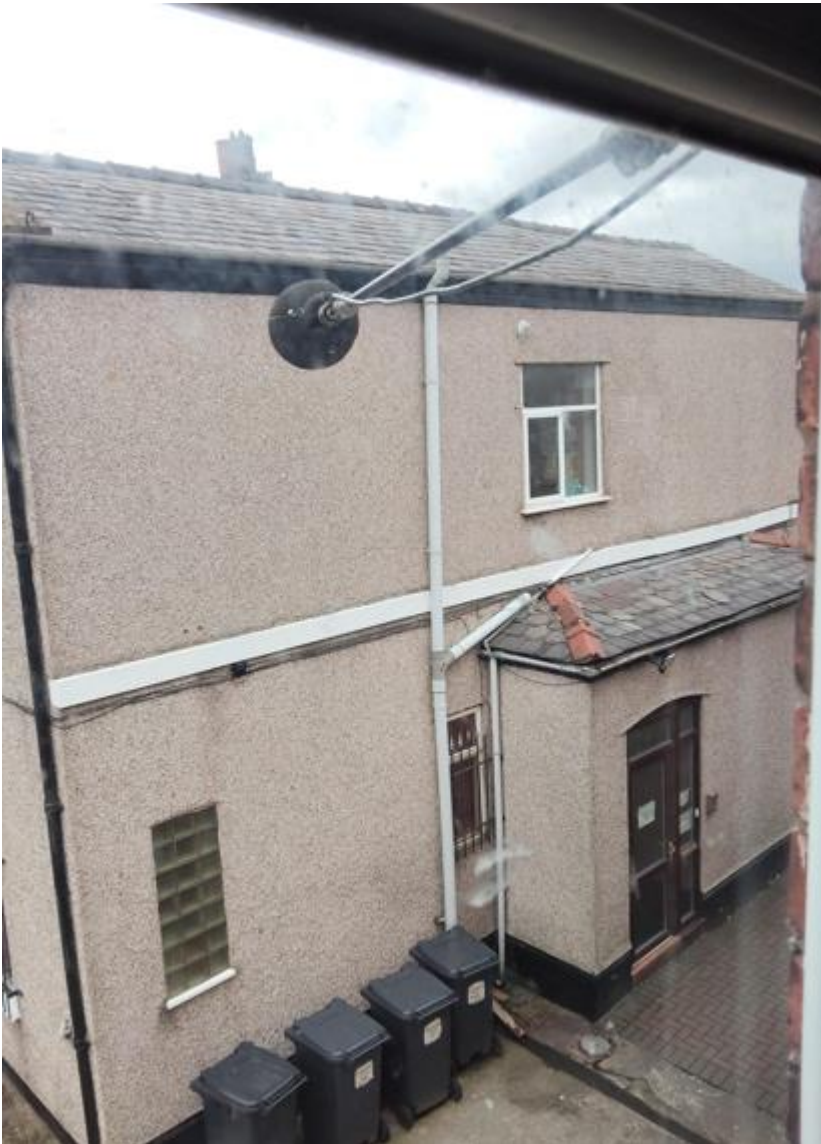
Figure 2: Photograph showing Monitoring Position 2
