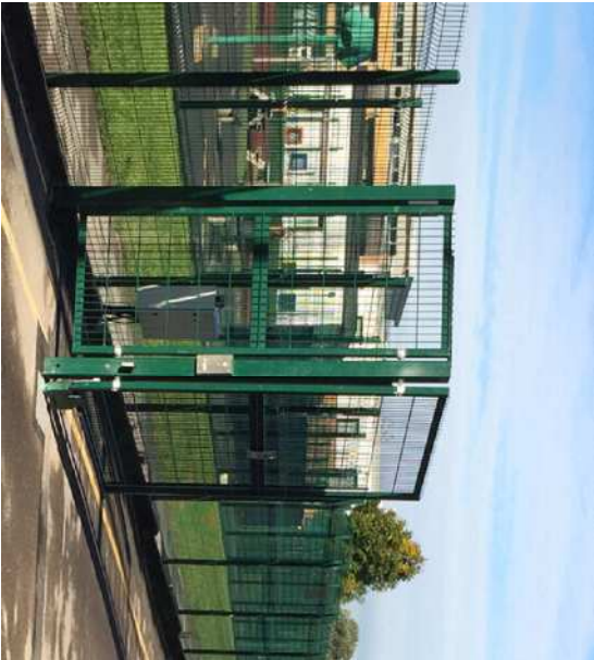
Typical style of new pedestrian gates to G1, G4, G5, G7 & G8 - All gates to be 2200mm to match fence height - width as per drawing ref: 2335_T_003
