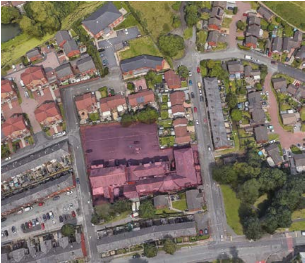
The site is located between Whittaker Street and Parsonage St, Radcliffe, Bury. A previous 2 storey red brick building occupied the site which was a former school building and in more recent times had been used as offices. with circa 56no. car and bus parking spaces accessed from Whittaker St. The surrounding area is predominantly residential, and the schoolshall be a key part of the local community. There is access to the site via the established vehicular and pedestrian access along Whittaker Street, and parking and delivery of materials will be managed to minimise disruption to local residents (refer to site analysis and photoagrahic study below).
