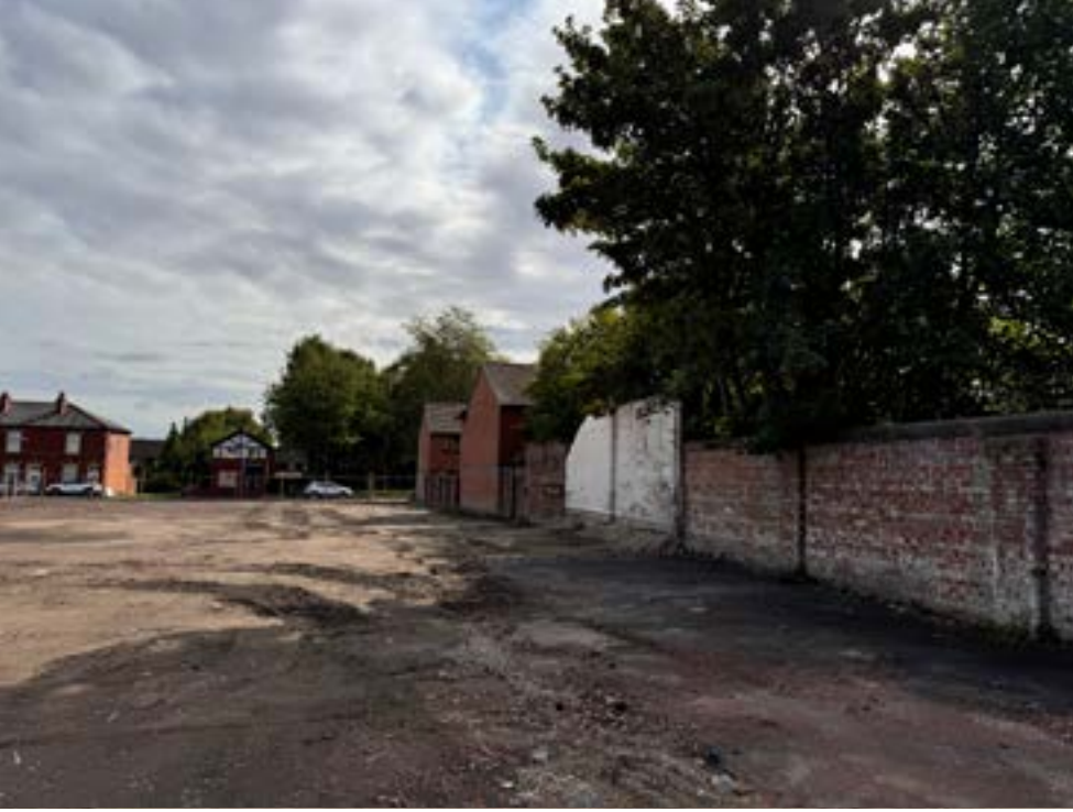
⑰ View within site towards southern boundary where new 2.4m high palidin fence shall be located.
