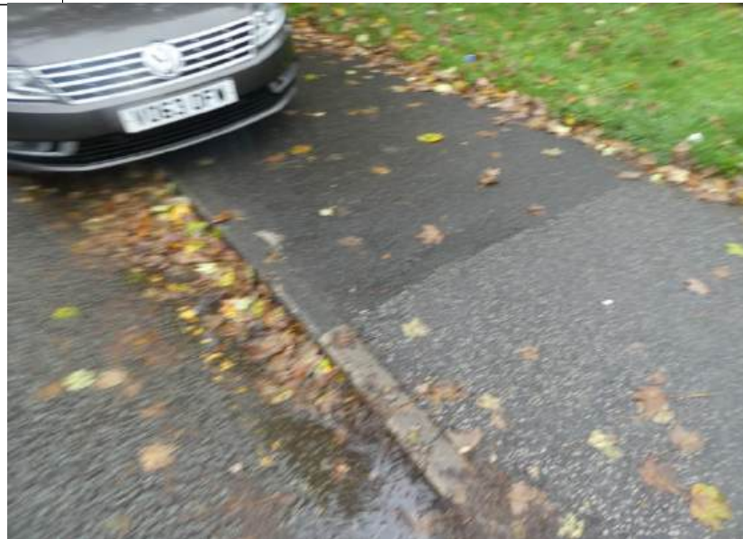
Photograph 72. Footpath in reasonable condition
