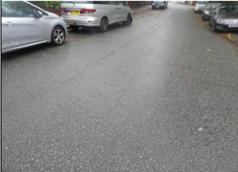
Photograph 71. Road surfacing in reasonable condition
