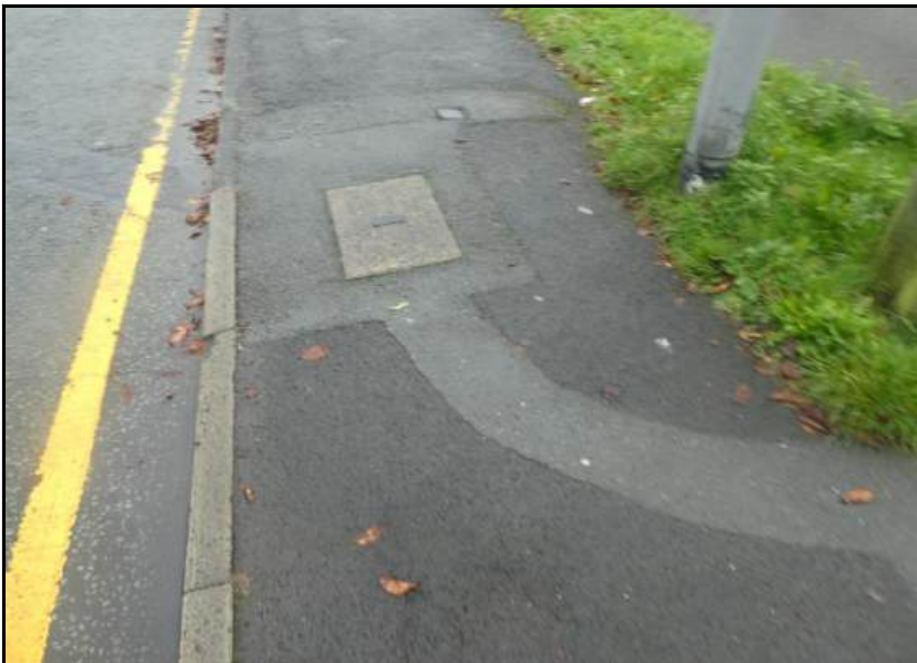
Photograph 65. Localised reinstatement to footpath
