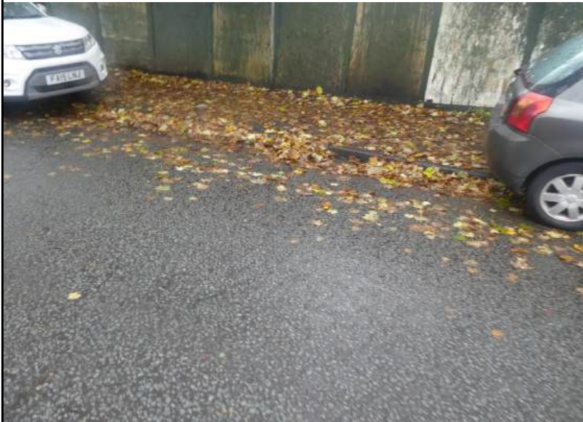
Photograph 75. Road surfacing in reasonable condition
