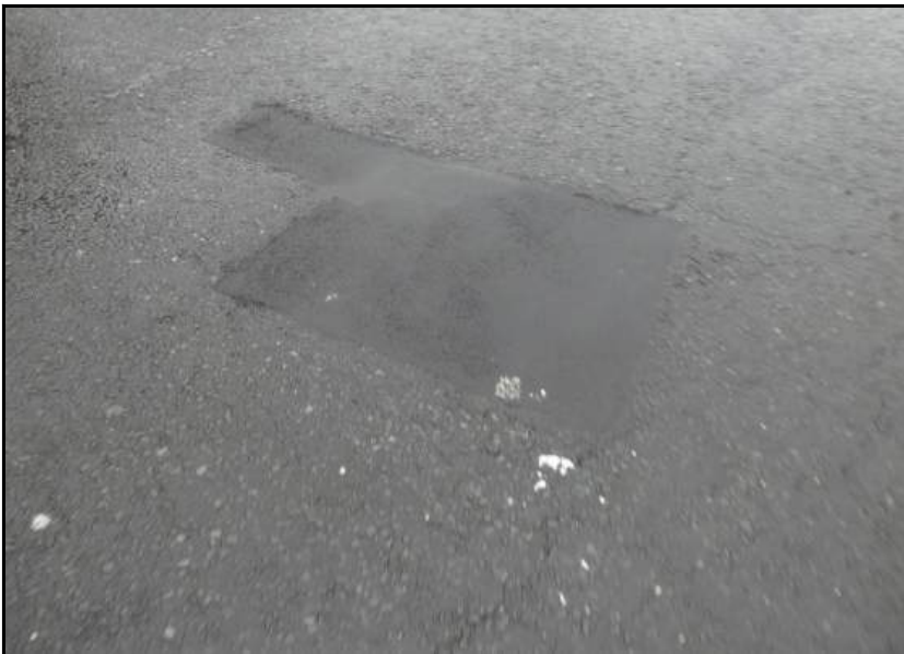
Photograph 85. Localised reinstatement of road surfacing.
