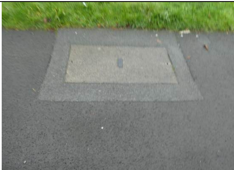
Photograph 66. Localised reinstatement to footpath
