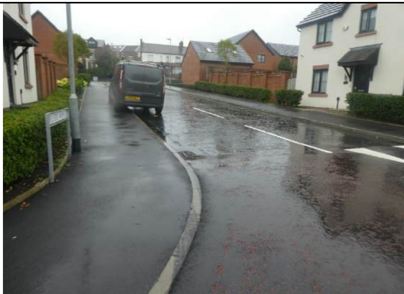
Photograph 2. Recently formed roadway and footpath surfacing
