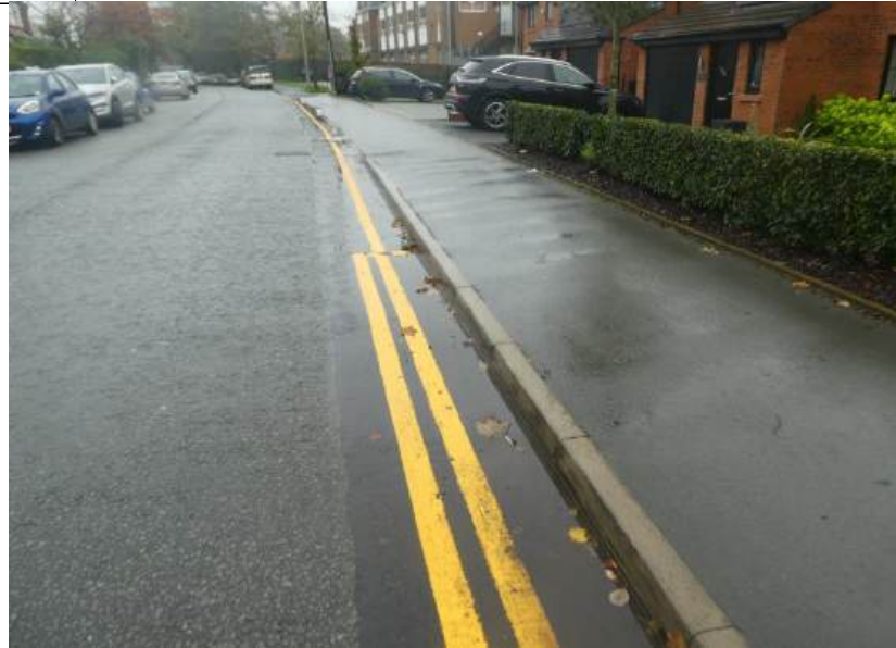
Photograph 56. Footpath in reasonable condition
