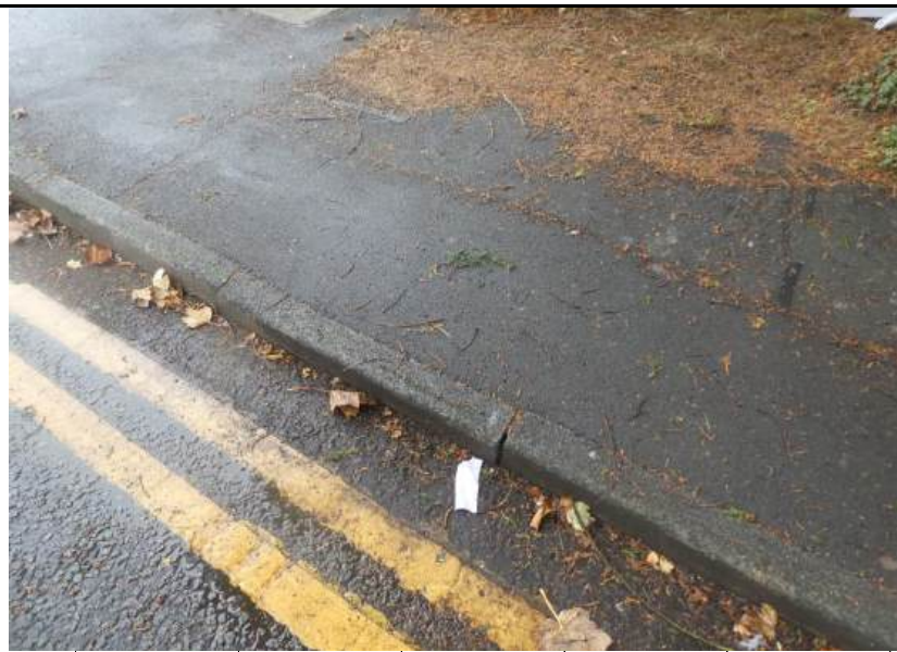
Photograph 42. Uneven kerbing.
