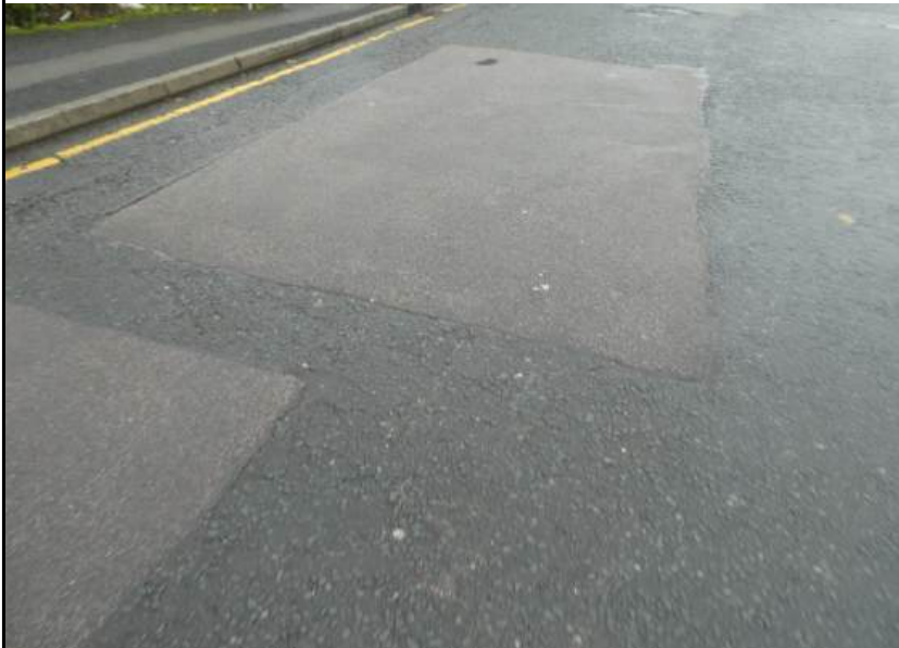
Photograph 87. Reinstatement of road surfacing.
