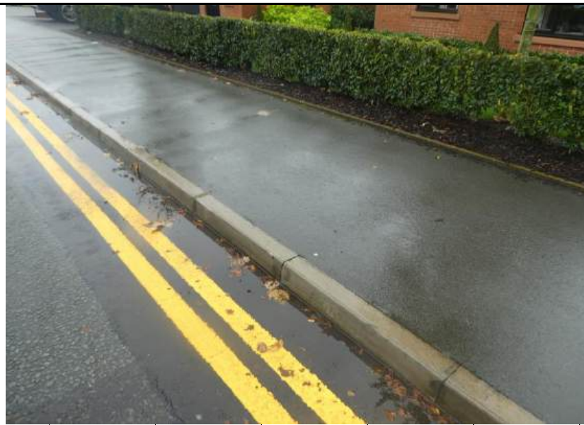
Photograph 54. Footpath in reasonable condition
