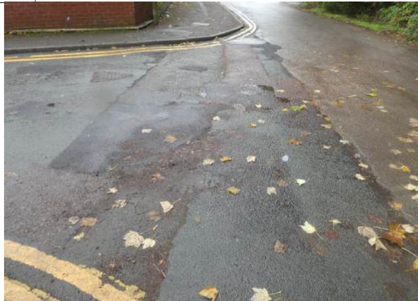
Photograph 16. Localised reinstatement of road surfacing to Norwood junction slightly eroded
