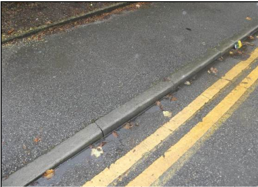
Photograph 29. Adjoining footpath in reasonable condition
