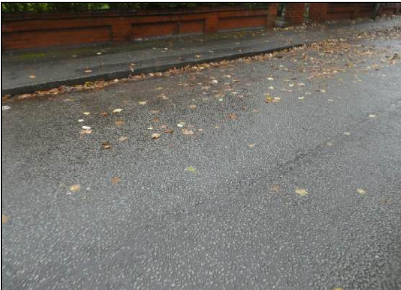
Photograph 73. Road surfacing in reasonable condition
