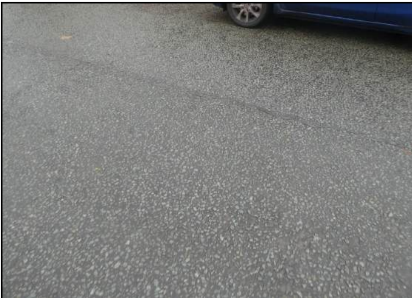
Photograph 57 Surfacing in reasonable condition.
