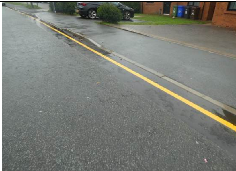
Photograph 58. Surfacing in reasonable condition.
