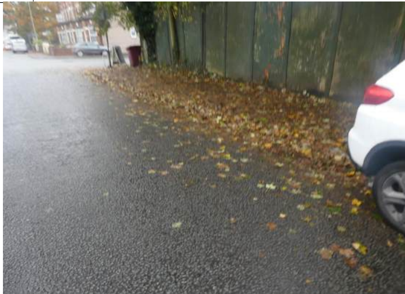
Photograph 76. Road surfacing in reasonable condition
