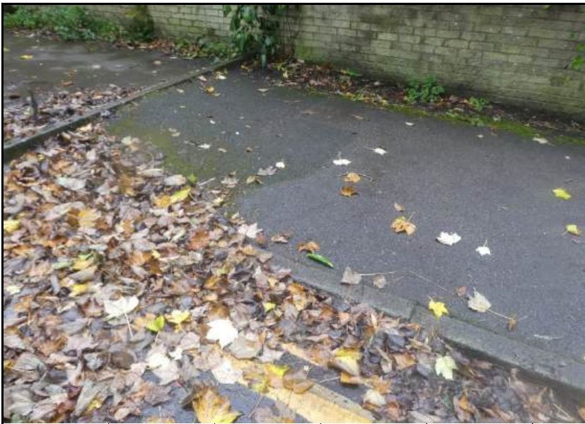
Photograph 13. Tarmacadam surfacing to the footpath
