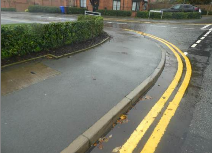
Photograph 55. Footpath in reasonable condition
