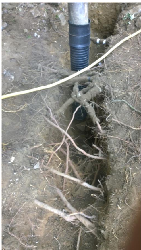
Plate 1: Use of Vacuum Excavator - Tree Roots protected by Hessian Wraps
