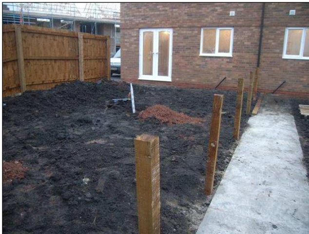
Photographs 13 and 14: Examples of validation photographs demonstrating validation hole location and soils forming inert cover
