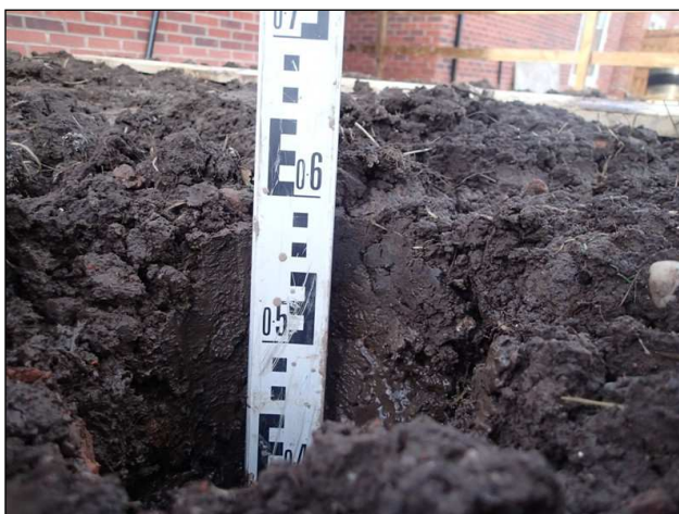
Photographs 15 and 16: Examples of validation photographs demonstrating inert cover depth and geotextile
