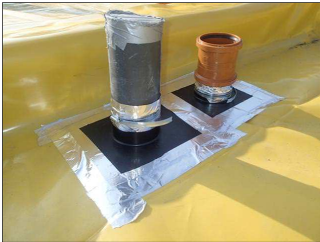
Photographs 24 and 25: Check tophat is sealed to membrane and pipework with tapes, and Jubilee clip
