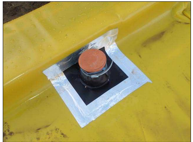
Photographs 24 and 25: Check tophat is sealed to membrane and pipework with tapes, and Jubilee clip
