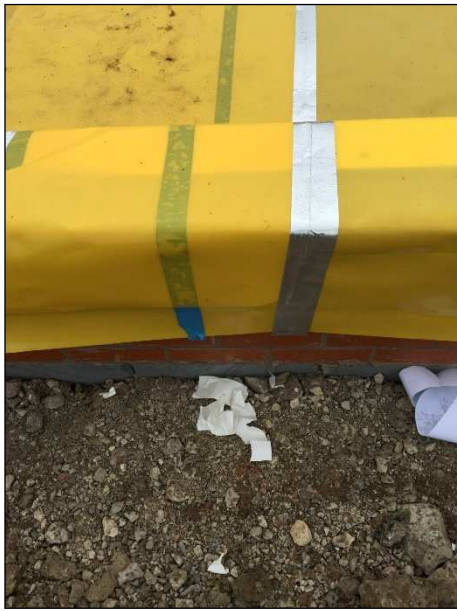
Photographs 22 and 23: Check >150mm overlaps of membranes and proprietary tapes placed and sealed with photographs taken
