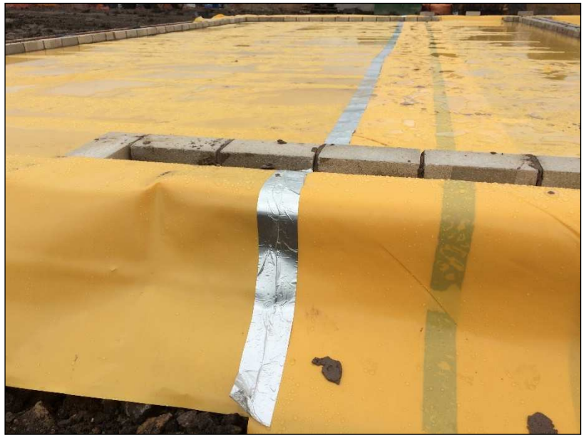
Photographs 22 and 23: Check >150mm overlaps of membranes and proprietary tapes placed and sealed with photographs taken
