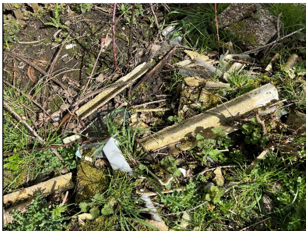
Photograph 7: Showing the presence of possible ACMs within the fly tipping present on site
