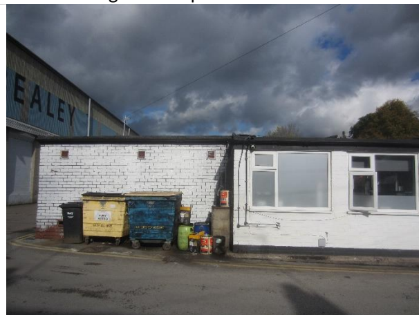
Photo 18: Western elevation of building B1
