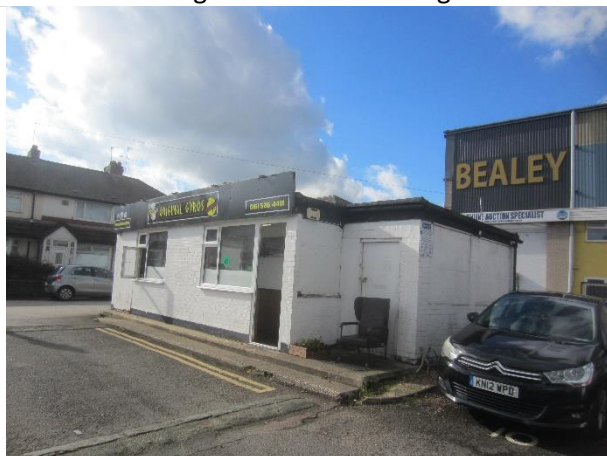
Photo 17: Southern elevation of building B1
