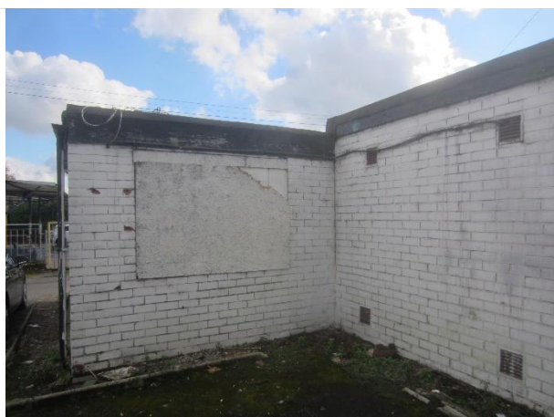
Photo 19: Northern and eastern elevations of building B1
