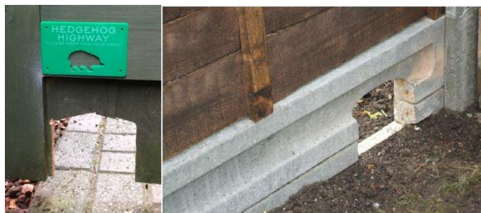
Insert 4: Showing wildlife access gap within fencing
