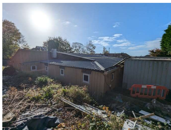
Photograph 6: Northwestern aspect of the pitched roof.
