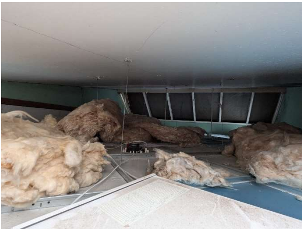
Photograph 8: Loft space over main building.
