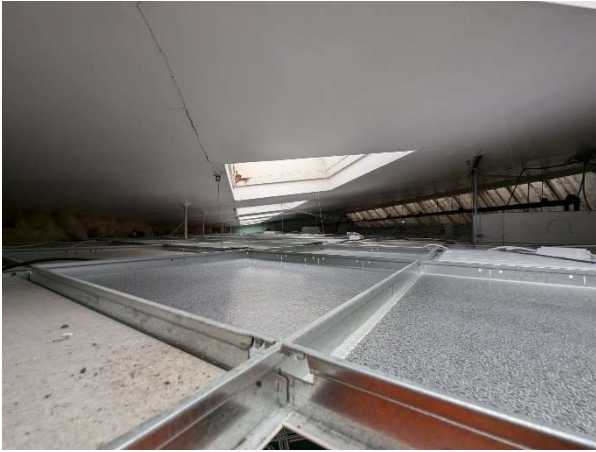
Photograph 7: Loft space over main building.
