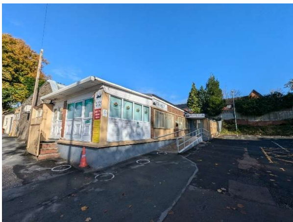
Photograph 1: Masjid-e-Bilal looking northwest.
