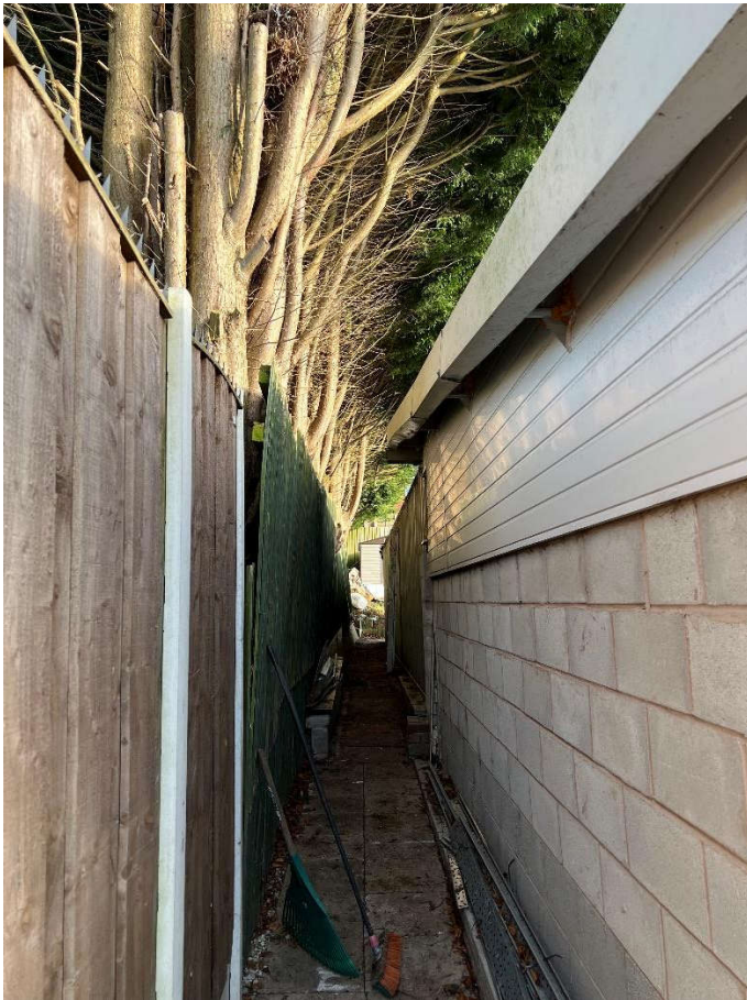
View alongside existing structure indicating overhang, poor historic pruning and displacement of fencing by incremental growth of stems /branches.
