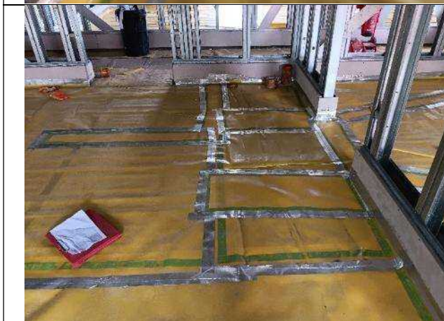
Photographs 7-10: Membrane coverage (including pathing / repairs)
