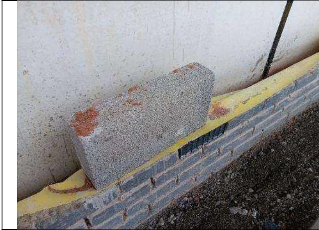
Photographs 11-12: Membrane lapped through wall cavity
