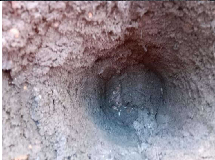
Photograph 2: View of cover system excavation in shared landscaping. Geotextile membrane present at base.
