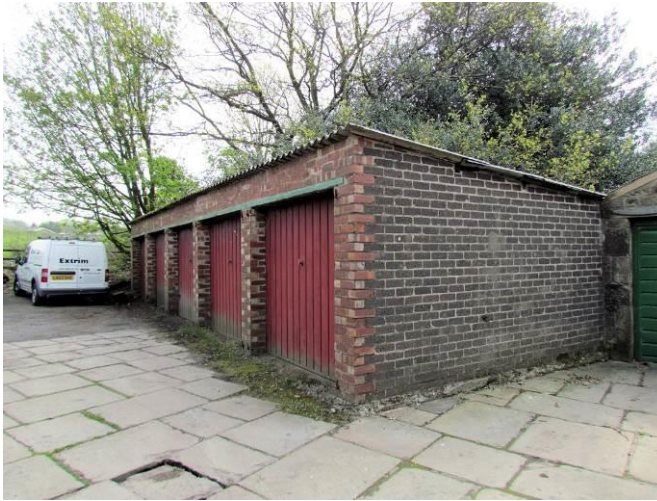
Late 20 th Century Brick Garages
