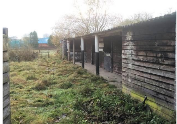
Stable Block to South-west
