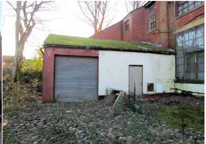
Added Garage and South Part of Rear Elevation
