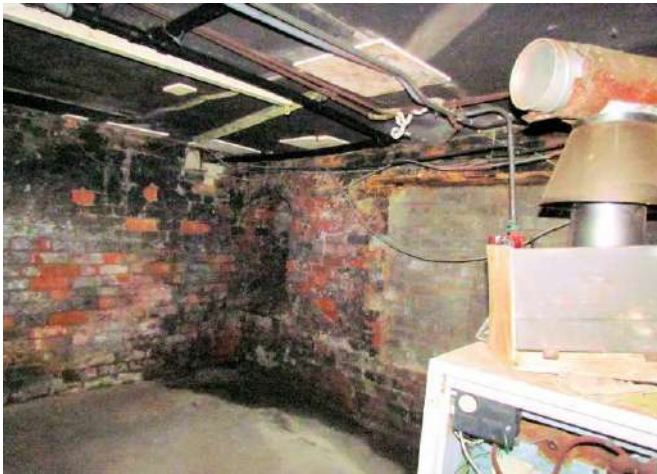
Room at North End of Basement
