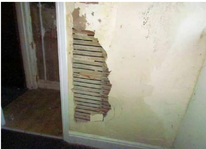
Collapsed Plaster
