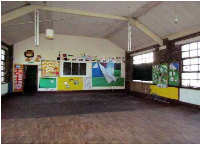
Northern Hall, Looking South
