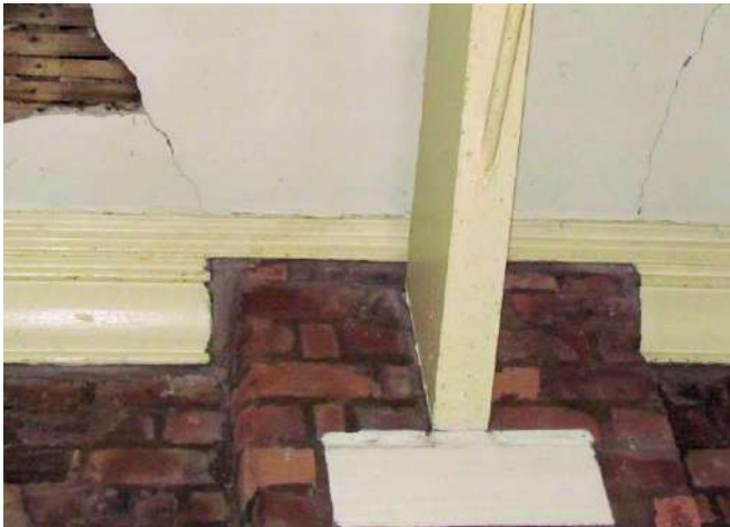
Detail of Cornice and Truss End
