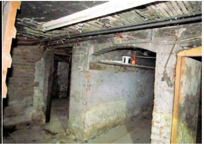
Northern End of Basement
