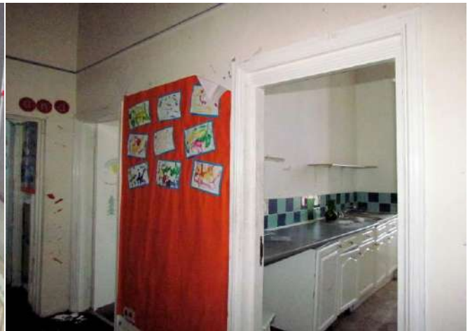
Historic Door Surrounds in Corridor
