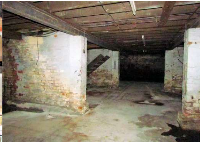
Southern Part of Basement
