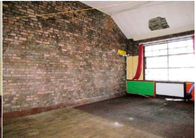
Southern Hall, Looking West
