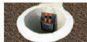
SGA Installed in Concrete Gully
