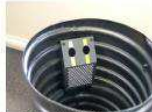
SGA Installed in Plastic Gully
