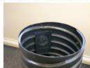
SGA Back-plate installed in Plastic Gully
