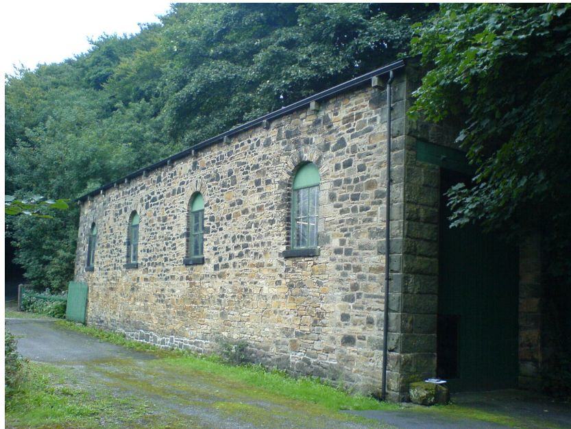
Engine shed viewed from the original sidings
