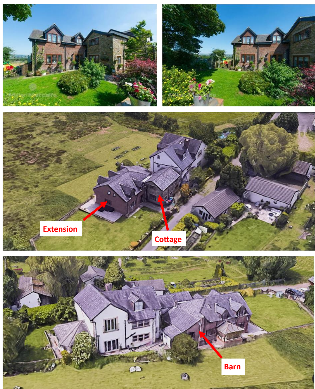
Image 4: Photographs of the existing property
