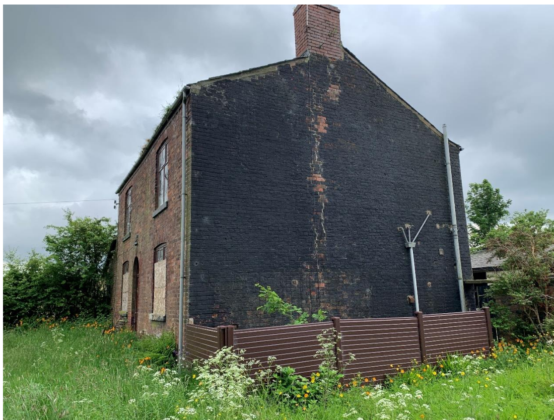
Plate 3 – The western elevation of the building
