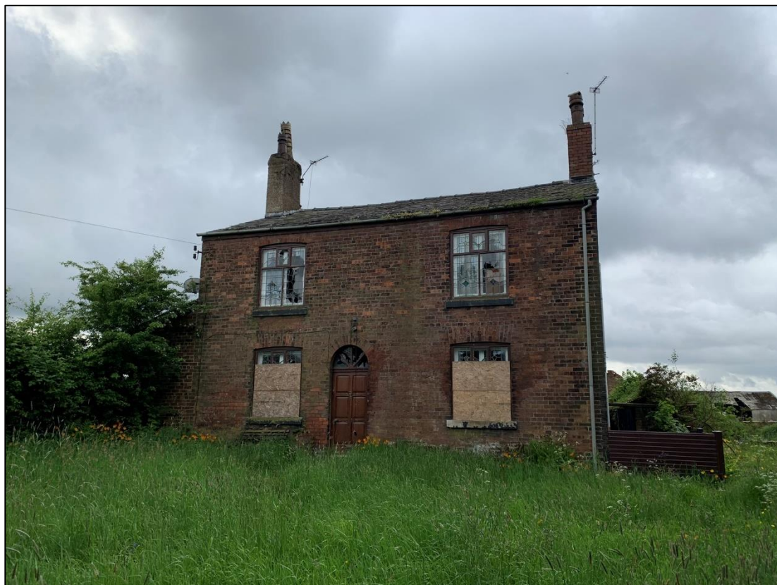
Plate 2 – The northern elevation of the farmhouse
