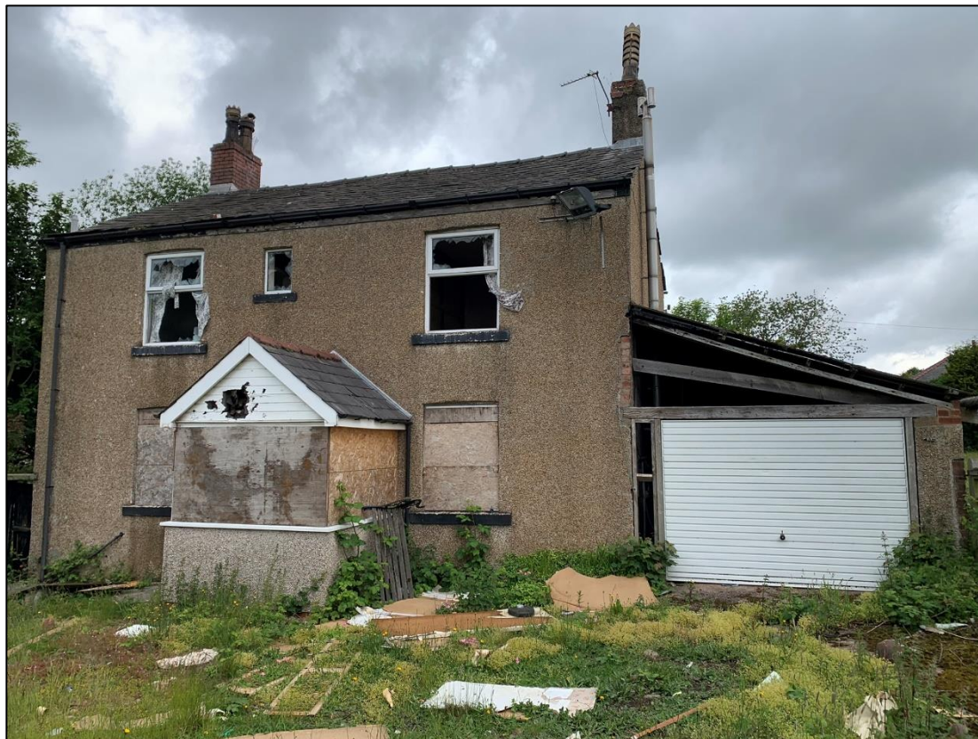
Plate 1 – The south elevation of the farmhouse
