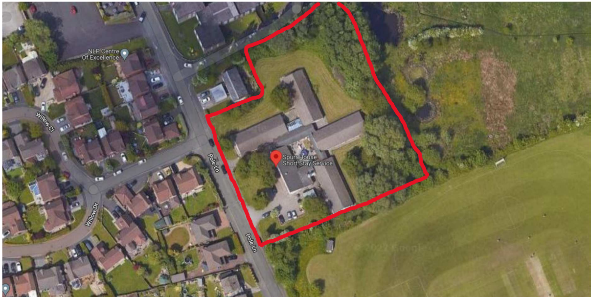
Fig.2 – An aerial view of the site
