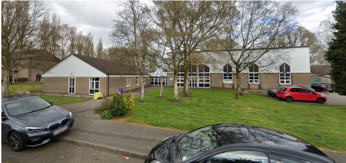
Fig 1 – The existing building frontage viewed from Pole Lane
