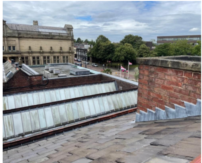
02 General view across the roofs, towards the new entrance. Note the weaving shed north-light roof and the art gallery in the background.
