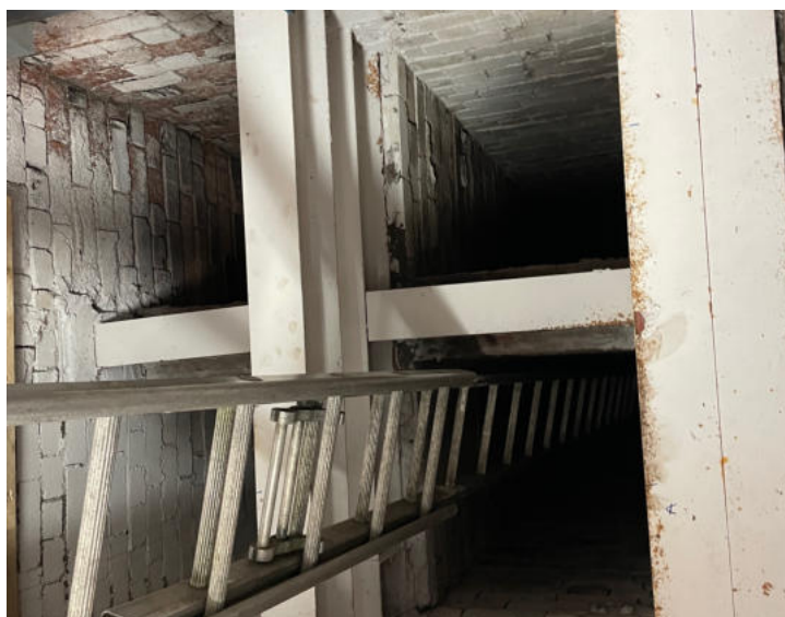
04 Internal view of the chimney/tower, showing the steelwork installed to support the brickwork separating the different flues (installed when a lift was installed)
