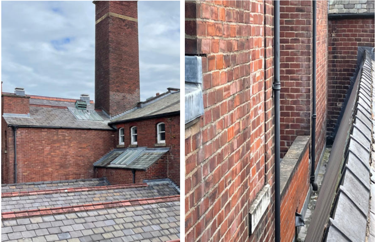
04 (Area G). General view (left). Close up of view of lead gutter, outlet from roof 11 (left).
