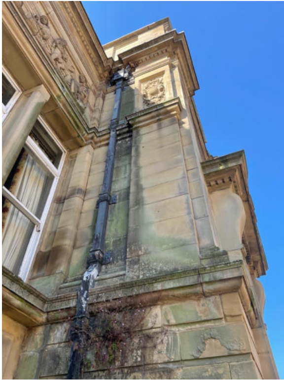
01 (Area A, right and B, left). Outlets and downpipes to Broad Street. Surcharging and discharging down the face of the ashlar. Causing damage to the stonework (externally) and damp internally. A combined cause of complex discharge arrangements at cornice level, lack of capacity and blockages can be identified as the causes.
