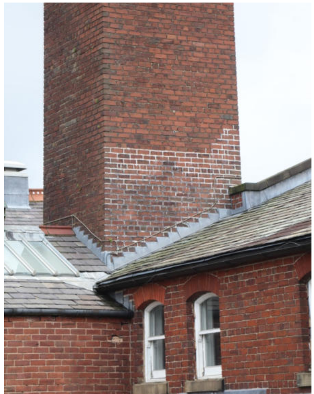
06 & 07 (Area D). Damage to finishes from water ingress above lift shaft (lift 1) and recent repointing works, which have made an improvement to the water ingress.
