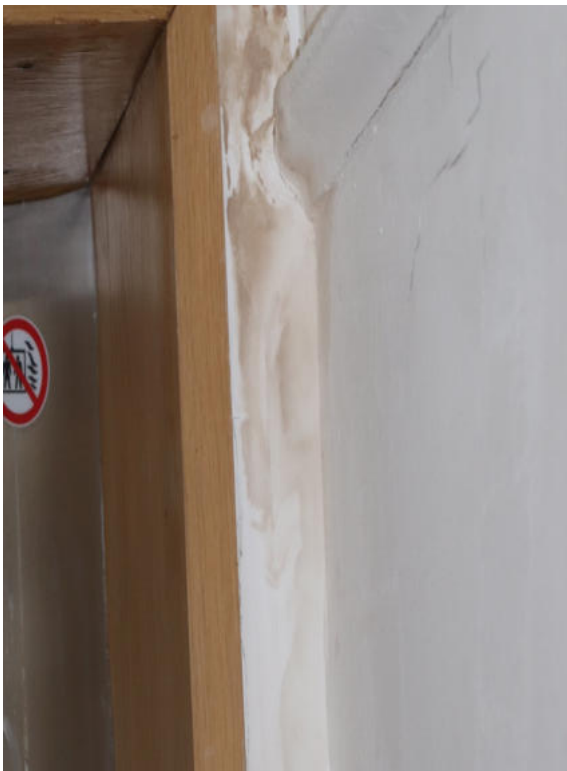
06 & 07 (Area D). Damage to finishes from water ingress above lift shaft (lift 1) and recent repointing works, which have made an improvement to the water ingress.
