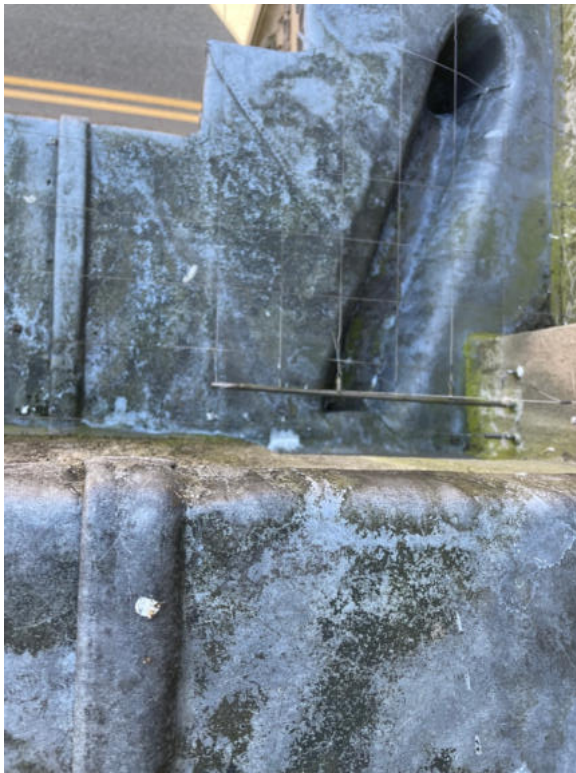
02 Area A (Note, Area B same but mirrored). Lead gutter discharges onto cornice, through channel cut into stone and lined in lead. Capacity is very limited and there is in effect no catch-pit or sump.
