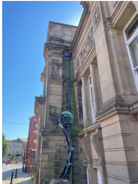
01 (Area A, right and B, left). Outlets and downpipes to Broad Street. Surcharging and discharging down the face of the ashlar. Causing damage to the stonework (externally) and damp internally. A combined cause of complex discharge arrangements at cornice level, lack of capacity and blockages can be identified as the causes.
