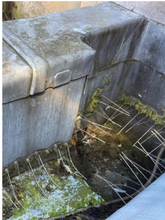
02 Area A (Note, Area B same but mirrored). Lead gutter discharges onto cornice, through channel cut into stone and lined in lead. Capacity is very limited and there is in effect no catch-pit or sump.
