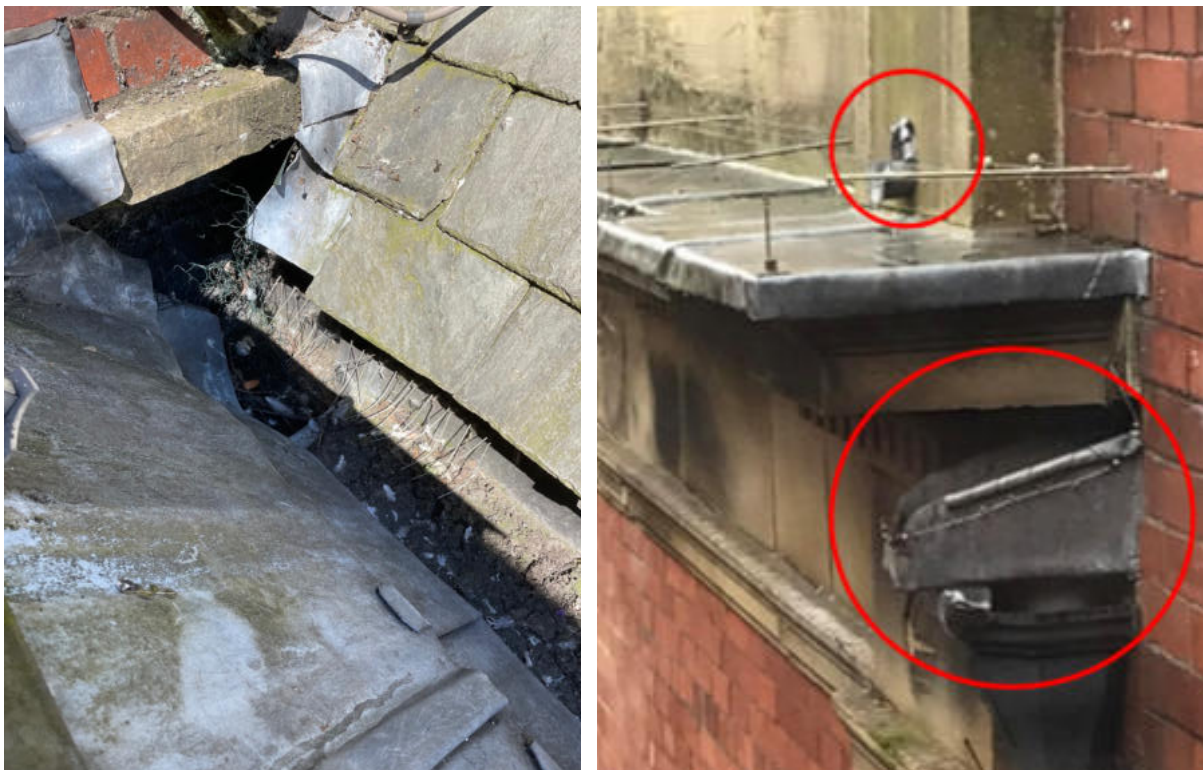
03 (Area C). View from the gutter above. View from the north-west showing the overflow and hopper (circled).
