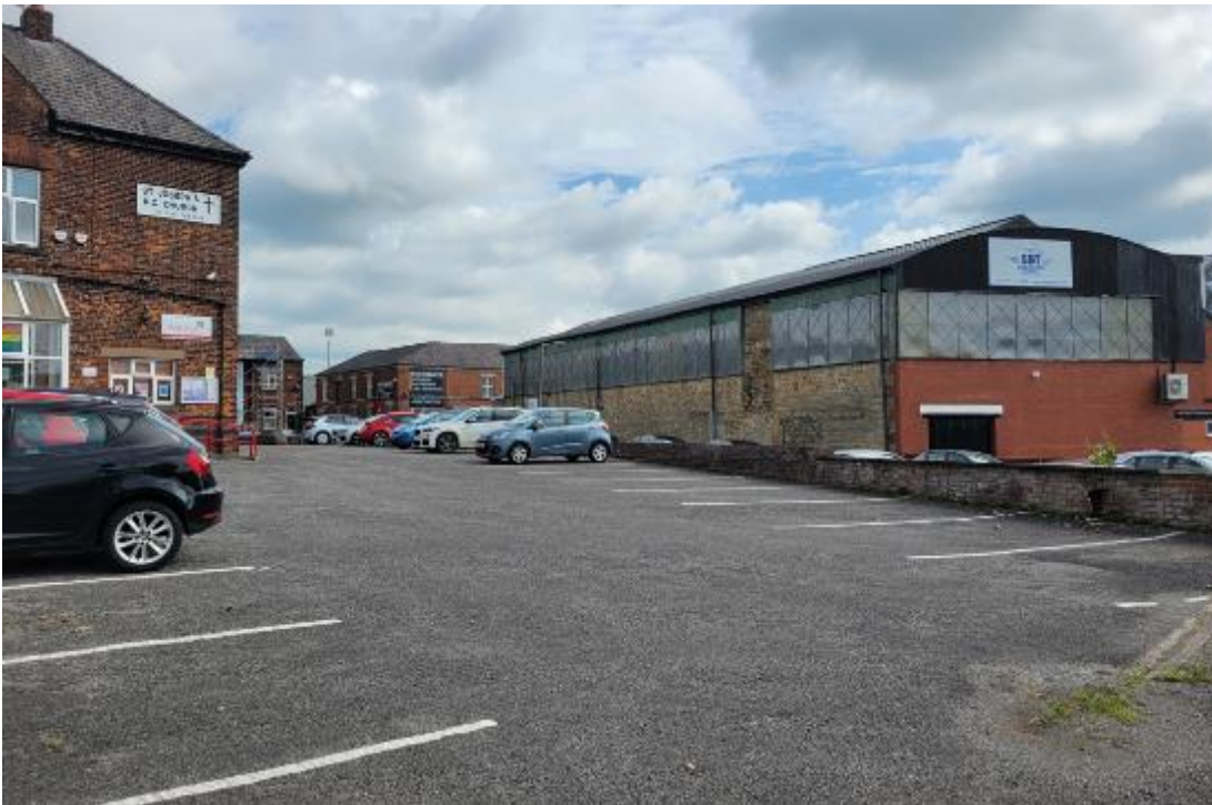
Plate B.3 Mortared wall present around the boundaries of the site
