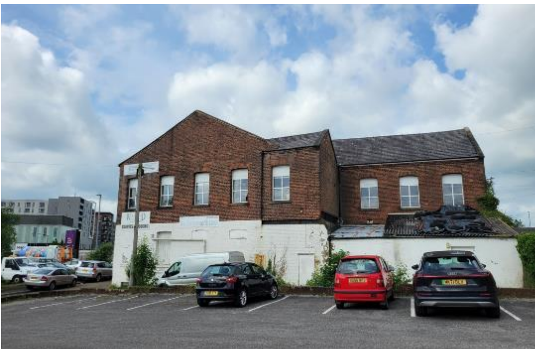
Plate B.4 Building B3 present adjacent to the site boundary, to the east
