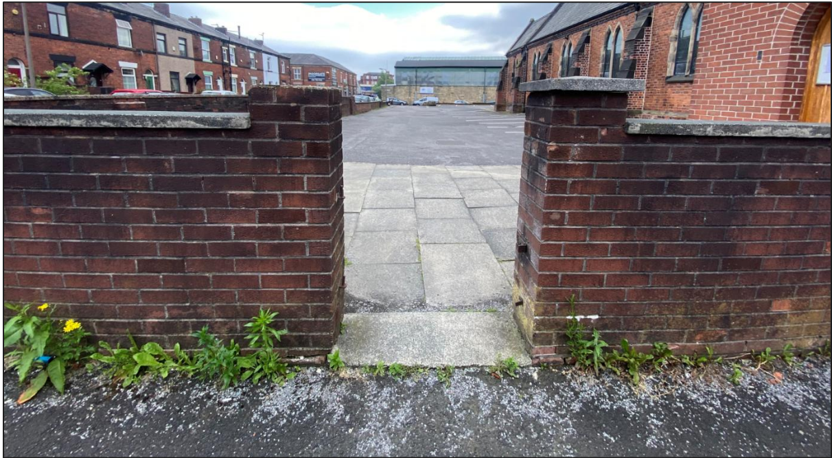
Photo 2.4: Pedestrian Access from Peter Street
