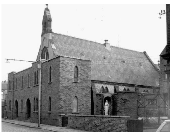
Figure 6: St Joseph's Church following the addition of the c.1950s two storey porch to the western frontage.
