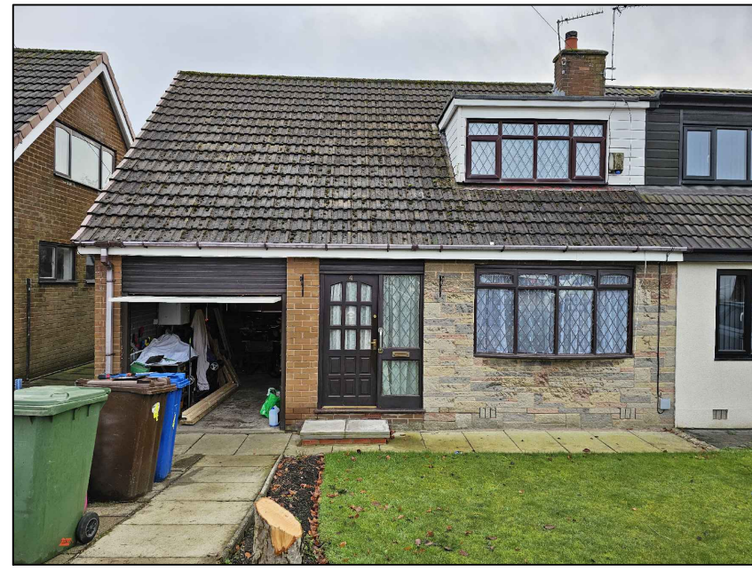
Site Photo-Existing Front Elevation
