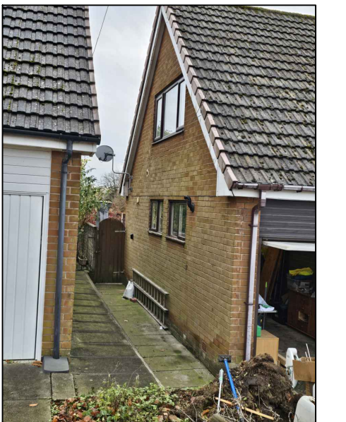
Site Photo-Existing Gable Elevation
