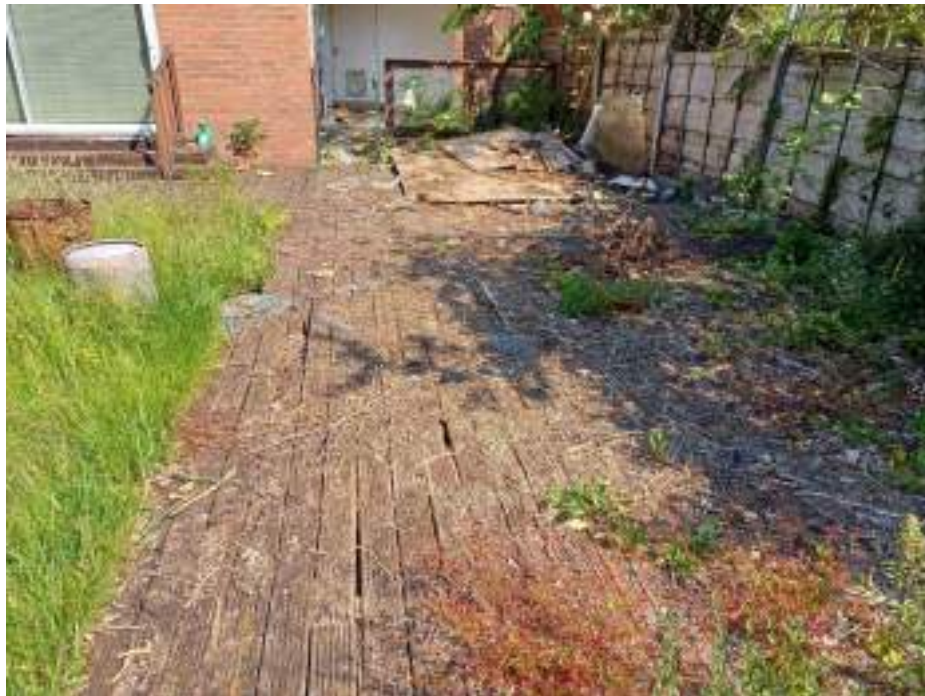
Photo 8: Remains of the shed structure in the southeast. No ACMs identified.
