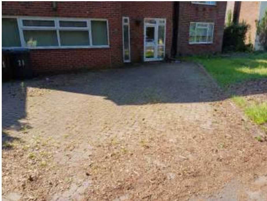
Photo 2: Parquet brickwork hardstanding at the front of the property, with a garden area to the west.
