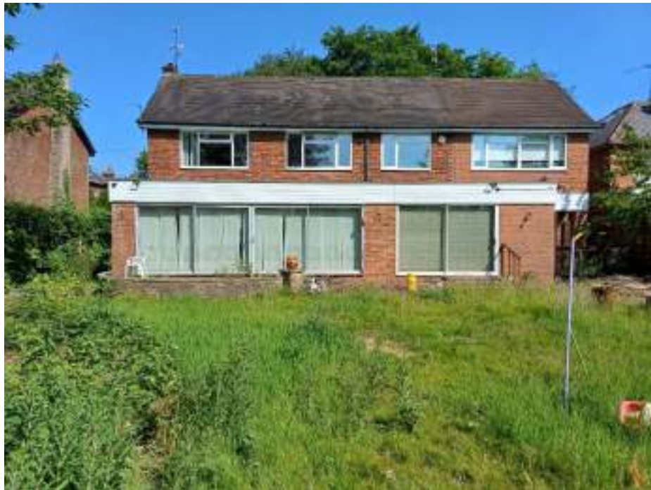
Photo 6: View of the rear of the property.
