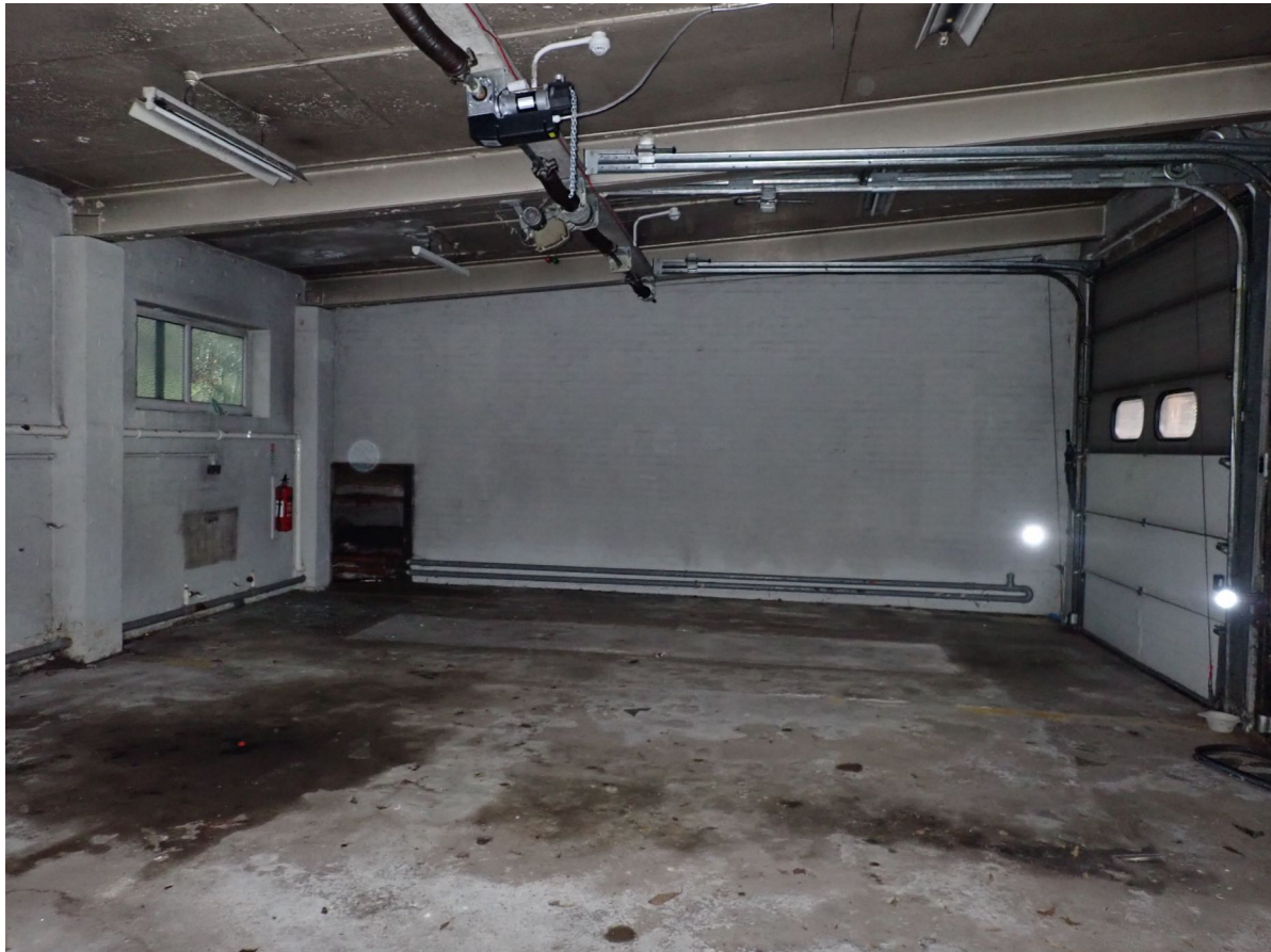
3.2a – Inside the ambulance bays.
