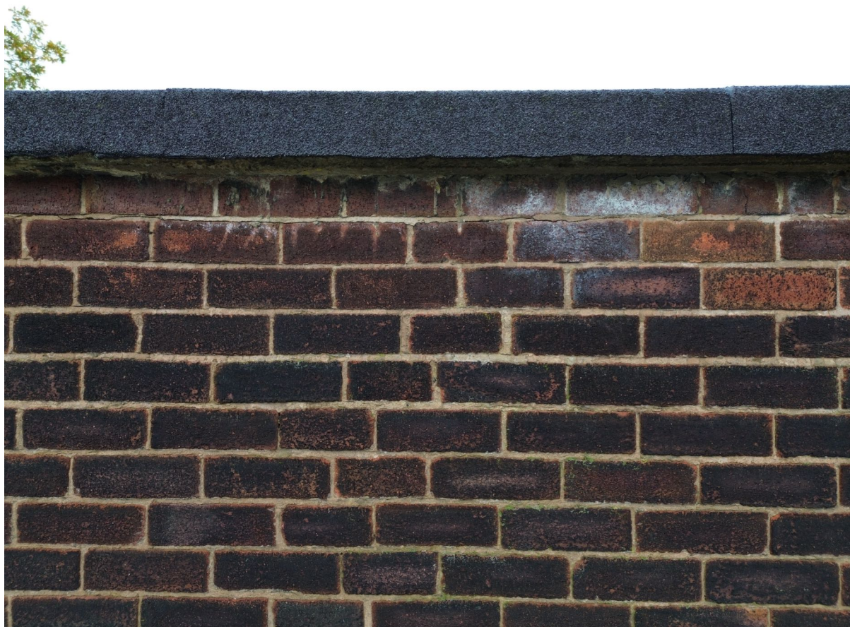
5 – There are no fascia boards at the eaves.
