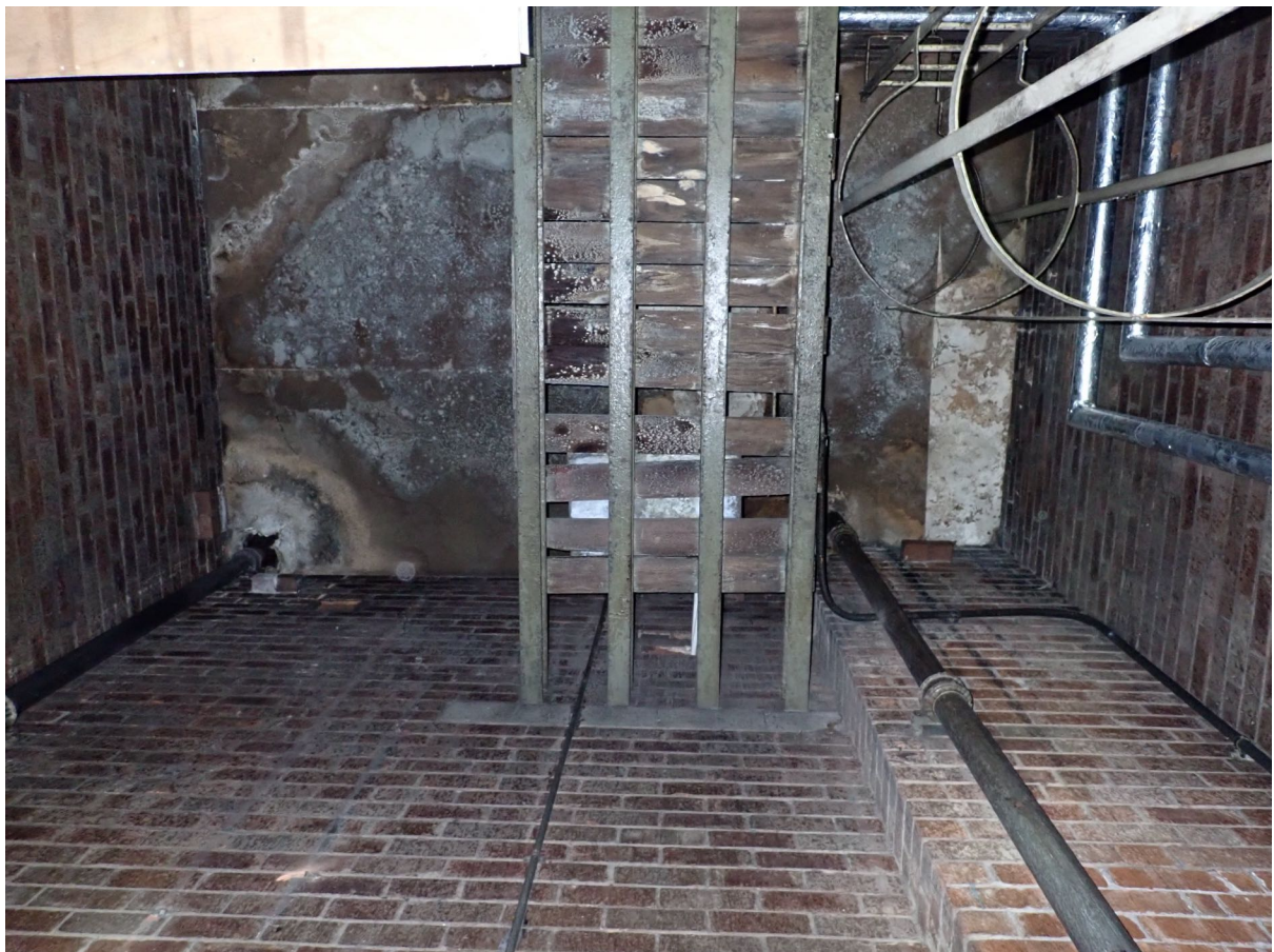
10 – The boiler room has bare brick walls, and a concrete roof.
