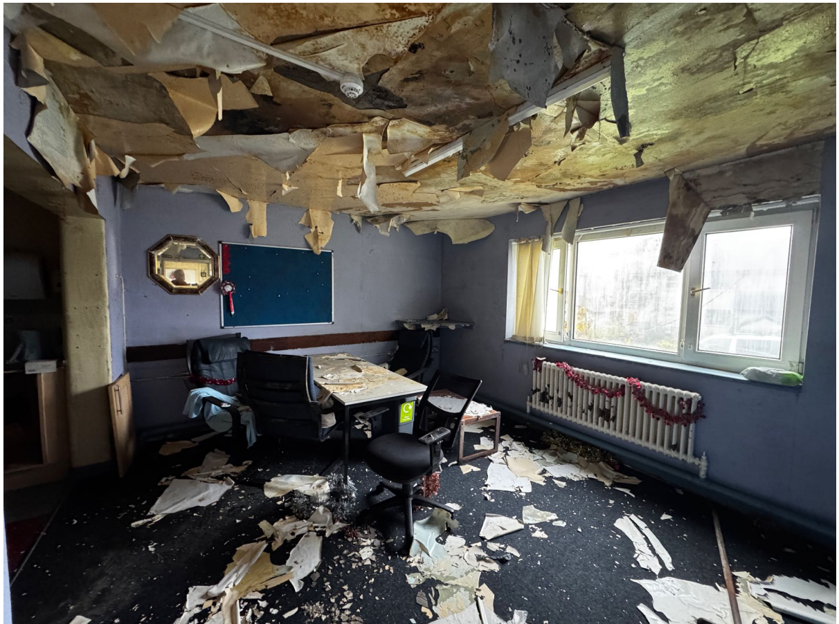
8 – Internally the offices are well lit by natural light and have been damaged by water.
