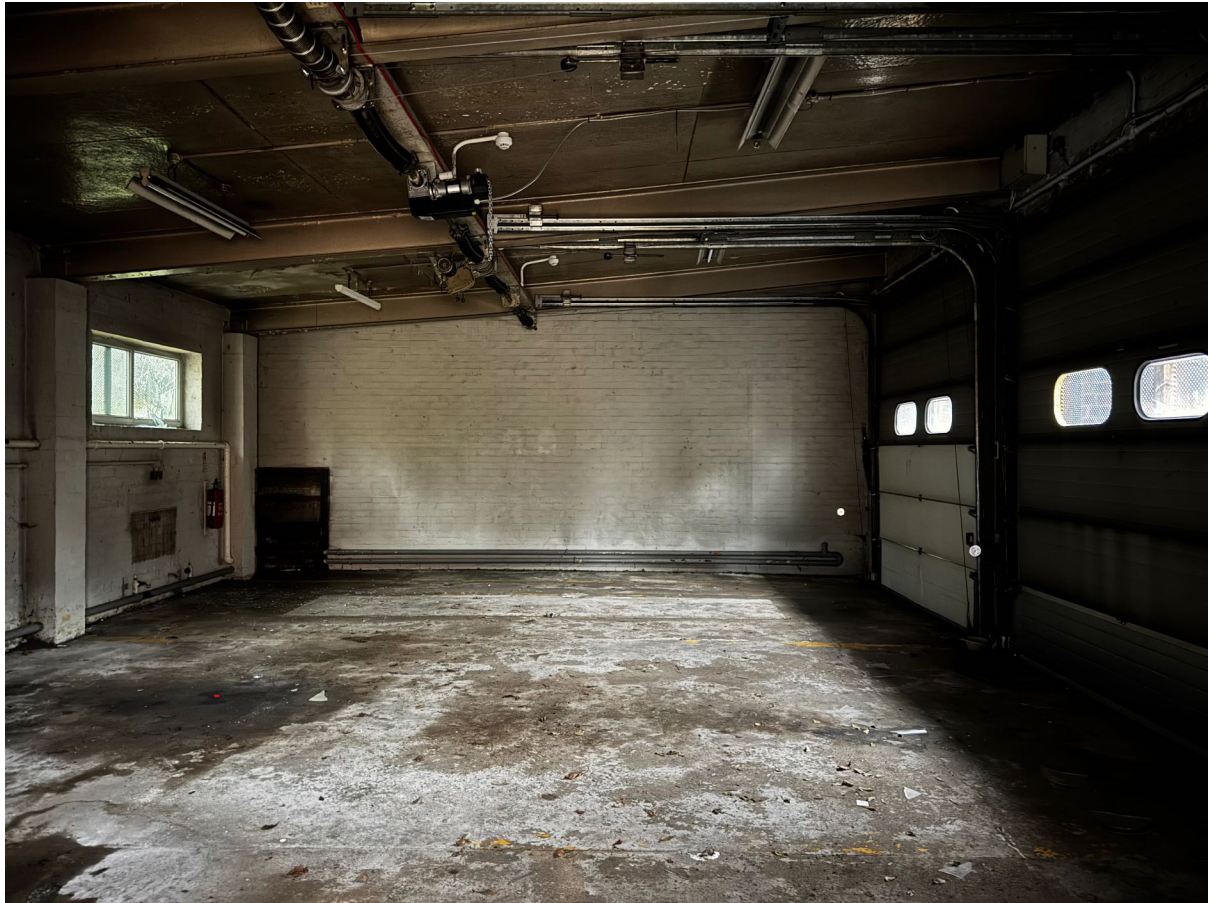
9 – The ambulance bays have painted brick walls with no roof void.
