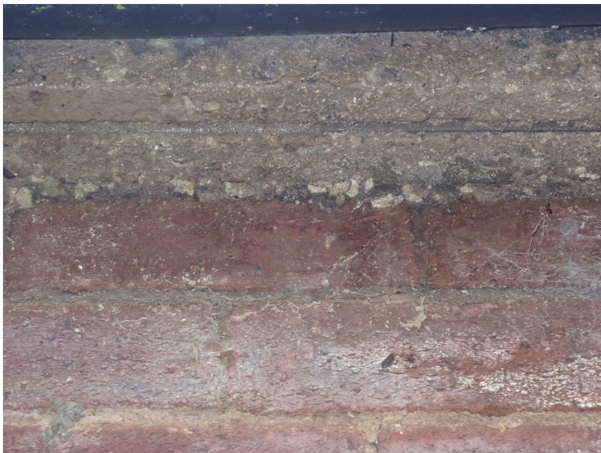
6 – There are no gaps between brickwork and the concrete roof.
