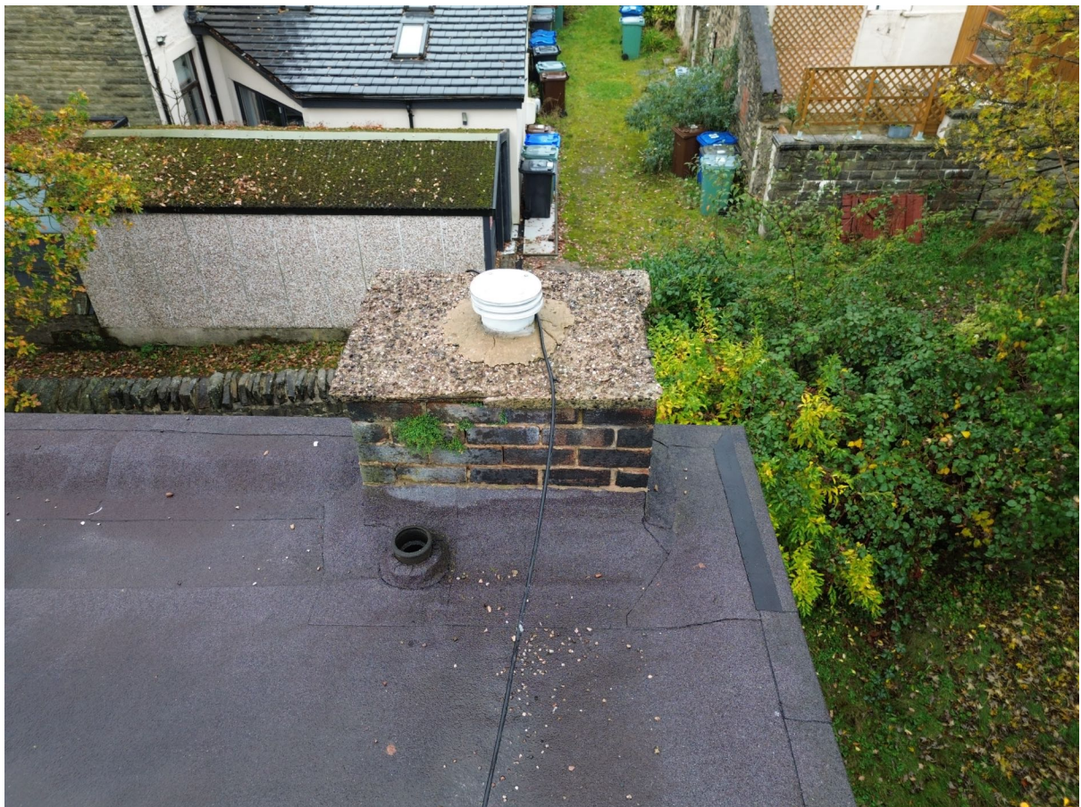
4 – Bitumen flashing is fitted tightly around chimneys and flues with no suitable gaps.
