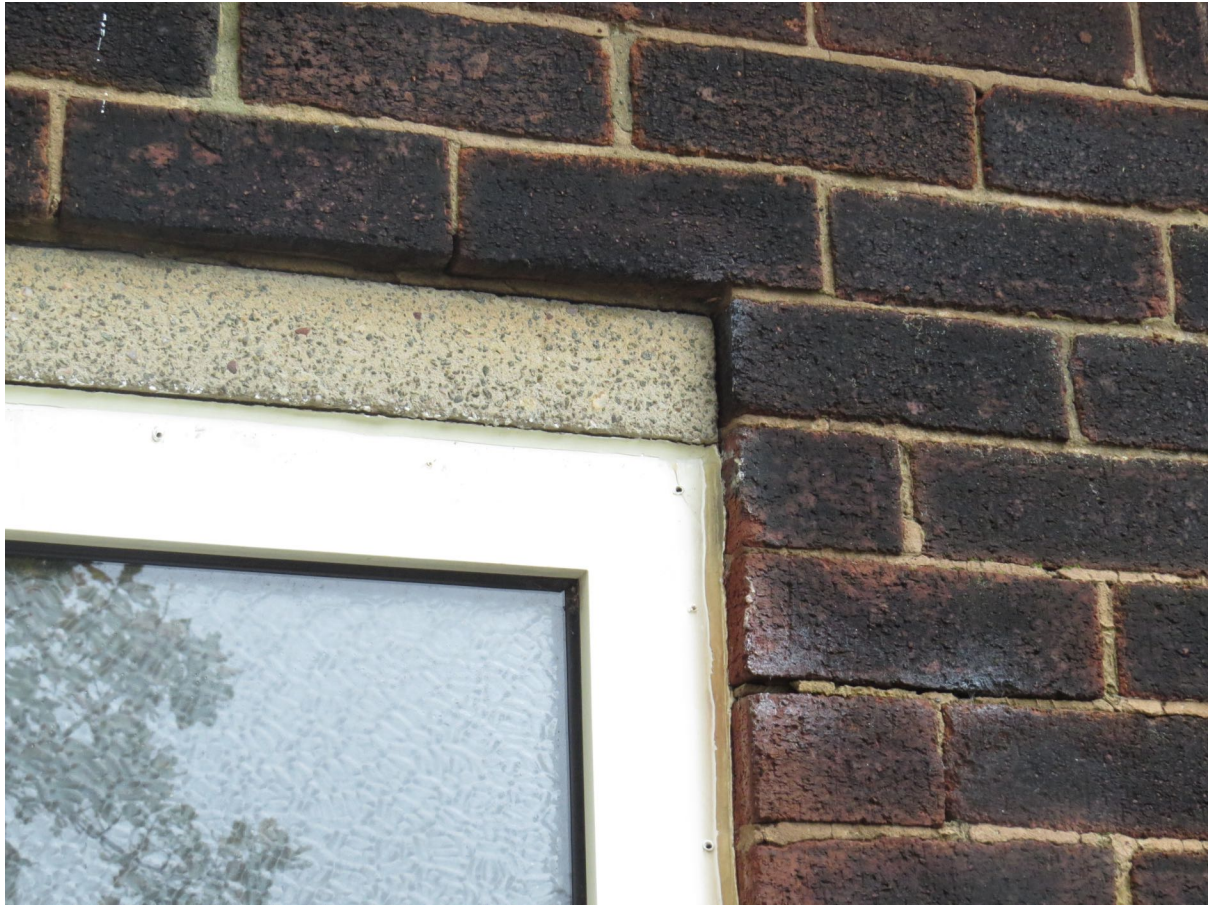
7 – Window and door frames are tightly sealed into walls with no suitable gaps.
