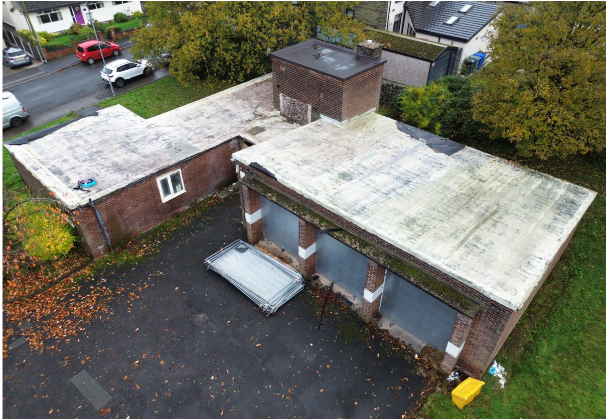
1 – The east side of the building.
