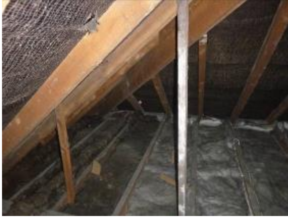
P1 Loft 1, insulated floor, felt lining
