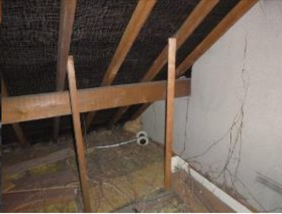
P2 Loft 2, insulated floor, felt lining
