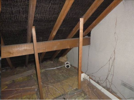
P2 Loft 2, insulated floor, felt lining
