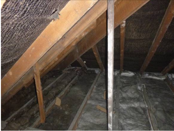
P1 Loft 1, insulated floor, felt lining
