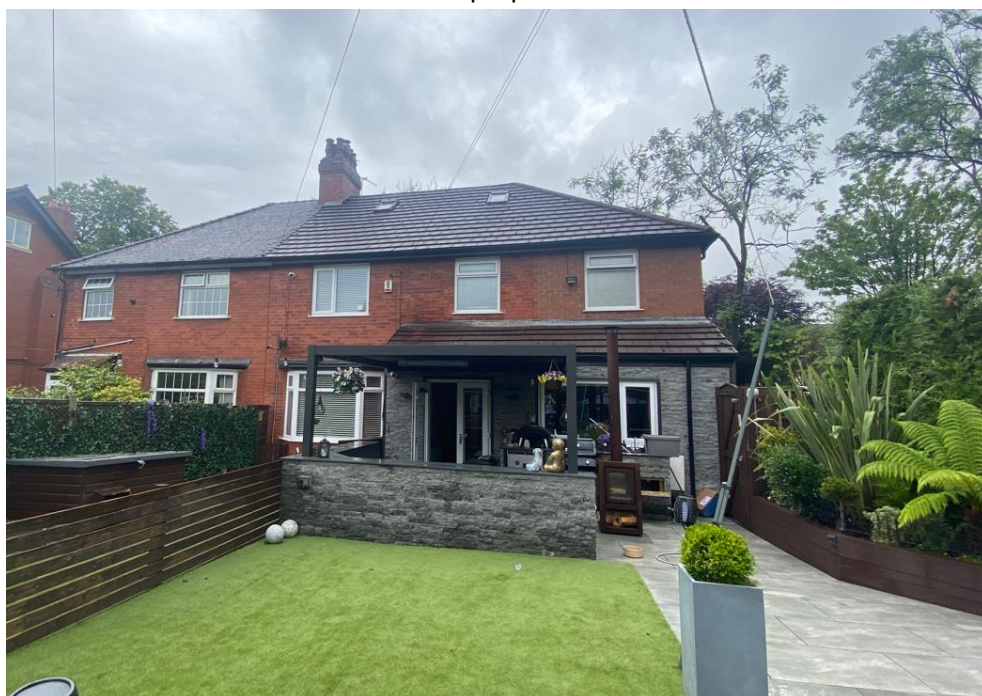
Photograph of the existing Rear House
