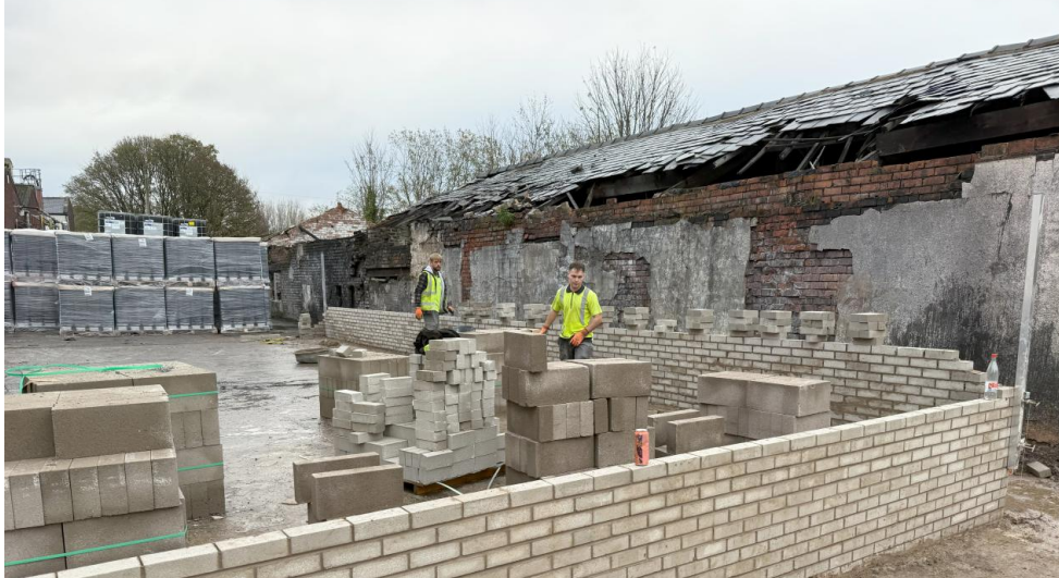
03. Commencement of masonry construction
