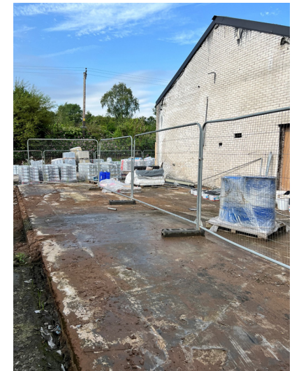
02. Existing slab retained after deconstruction of building following fire
