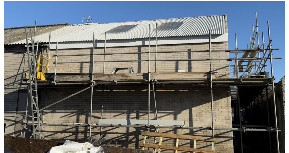
06. External view of roofing sheets and rooflights installed
