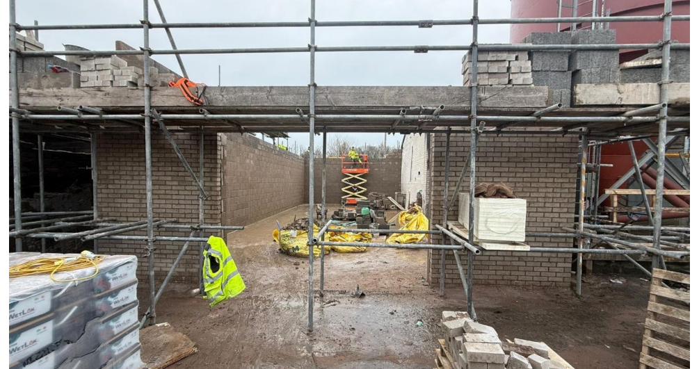
04. View of the front elevation showing structural opening for roller shutter
