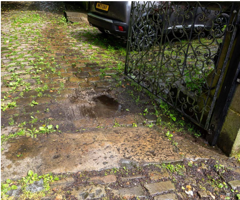
3 entrance gate threshold
