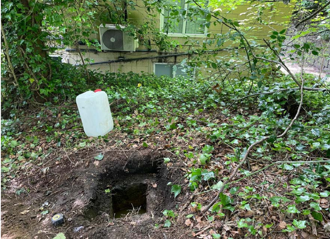
Photograph 5 – The pit was located in the south end of the site, in the location of a proposed courtyard.
