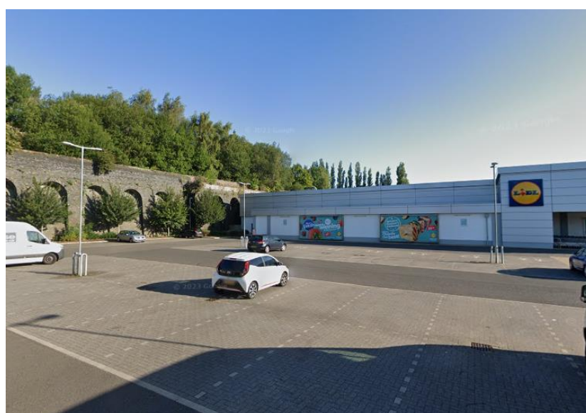
Figure 2. The site features a generous parking area shared with the adjacent Lidl
