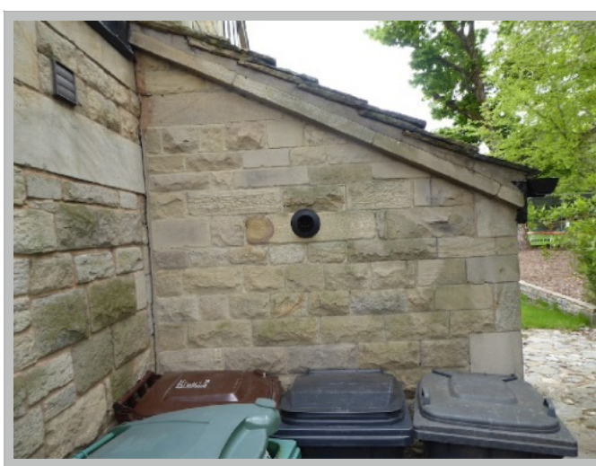
Plate 14. Extension on NW elevation, not keyed in
