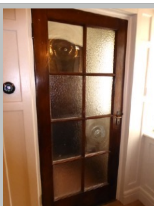
Plate 20. Glazed oak lobby door
