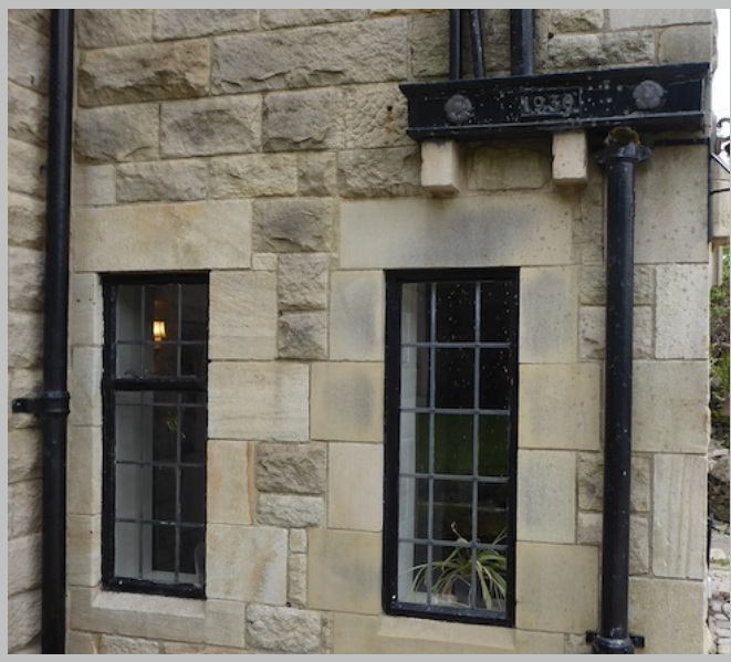
Plate 5. Metal framed windows and Hopper head with date 1930
