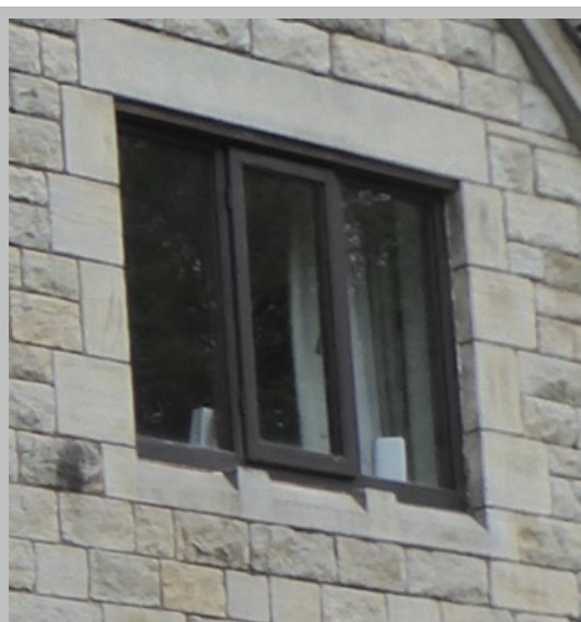
Plate 11. Window cills with bases for missing mullions
