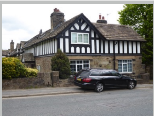
Plate 25. Front range of (Former) Bassfield Farm
