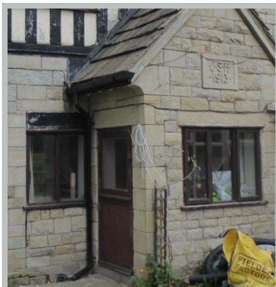
Plate 10. Porch, inserted and blocked doorway
