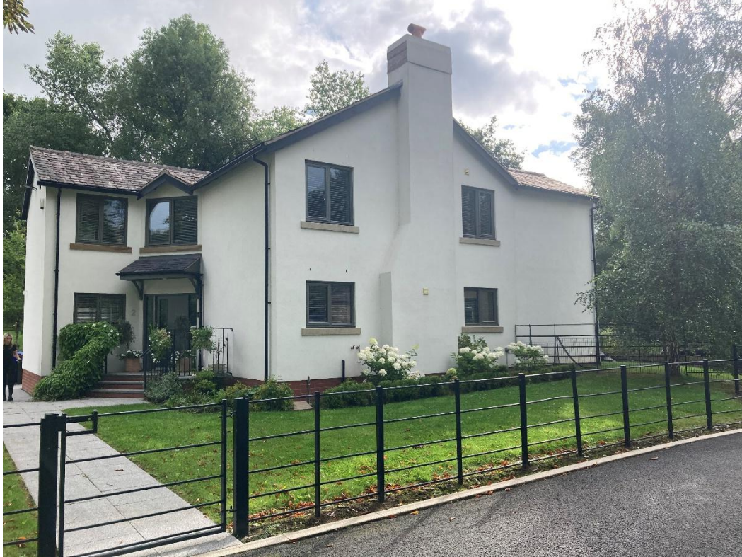
Image 1: Front elevation of 2 The Island
