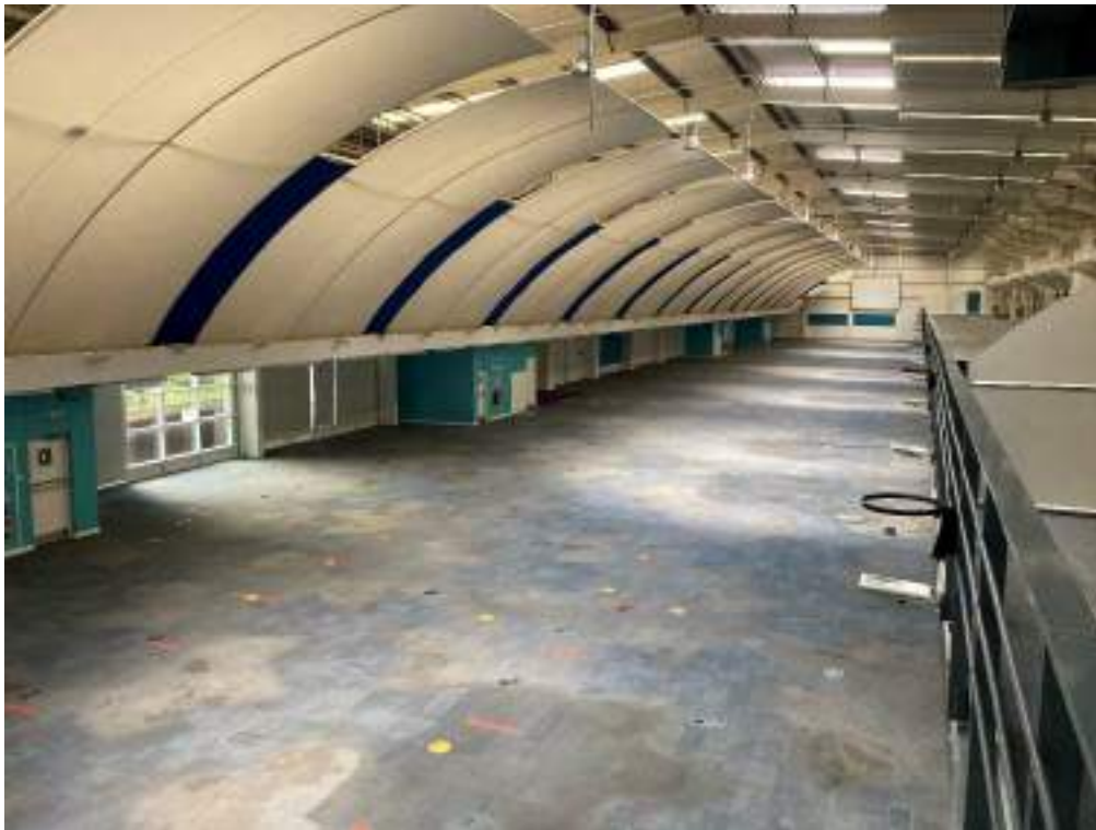
Photograph 9 - Open space area from single storey mezzanine (southern side)
