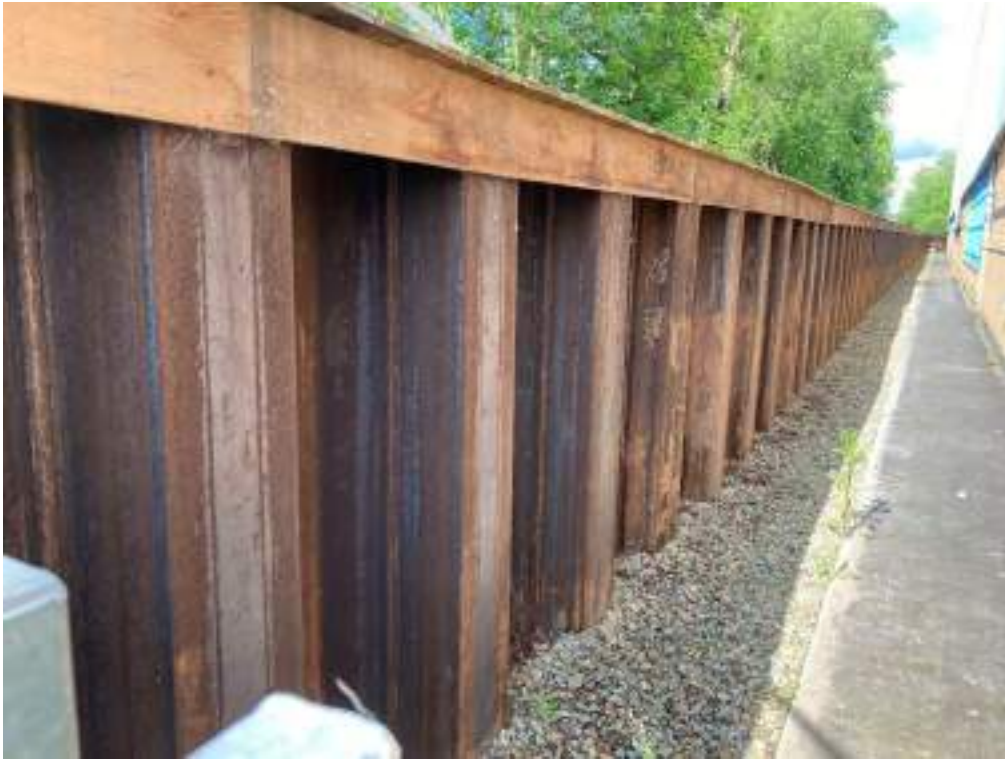
Photograph 3 - Sheet pile retaining wall structure (southern boundary)
