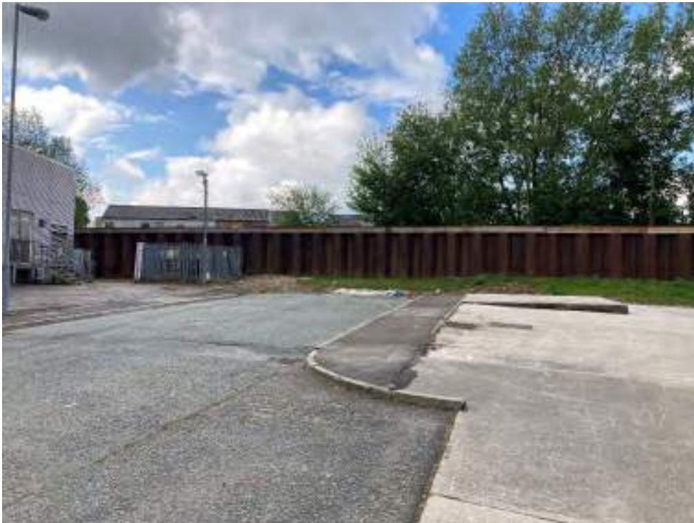
Photograph 4 - Sheet pile retaining wall structure (south-western boundary)
