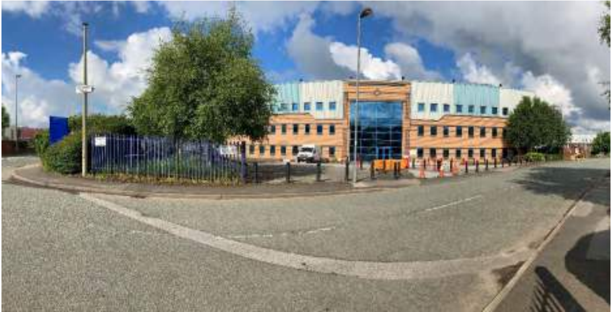
Photograph 1 – Building entrance (from unnamed road) and carpark.
