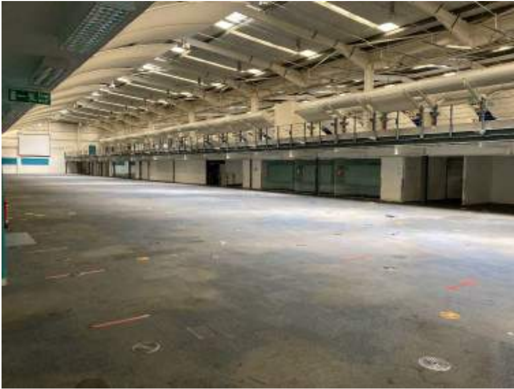
Photograph 11 – Single storey mezzanine from ground floor
