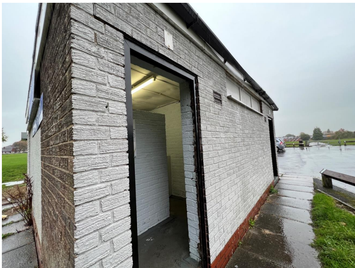
Photograph 4: The south elevation of the extension (toilet block).
