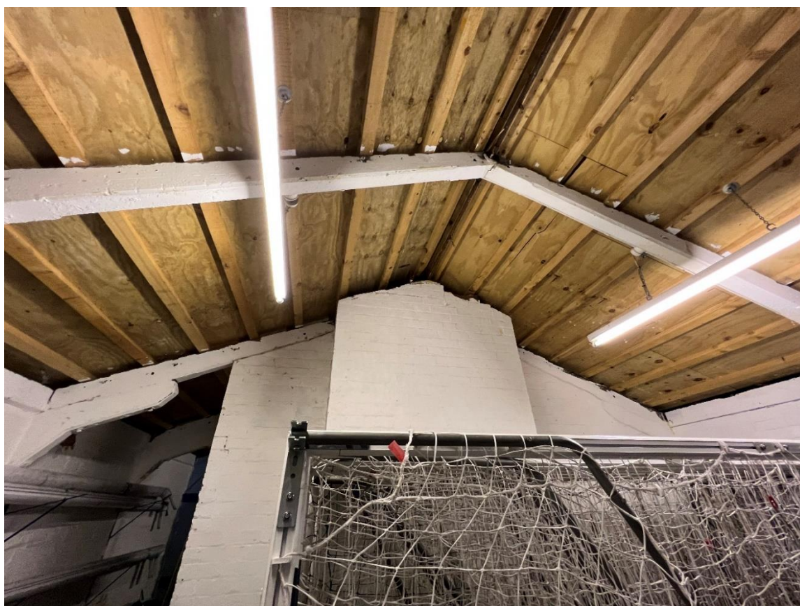
Photograph 5: Internal roofing structure of the changing area.
