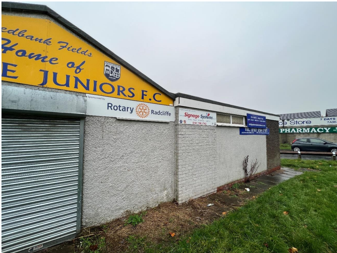
Photograph 2: The west elevations of the building.
