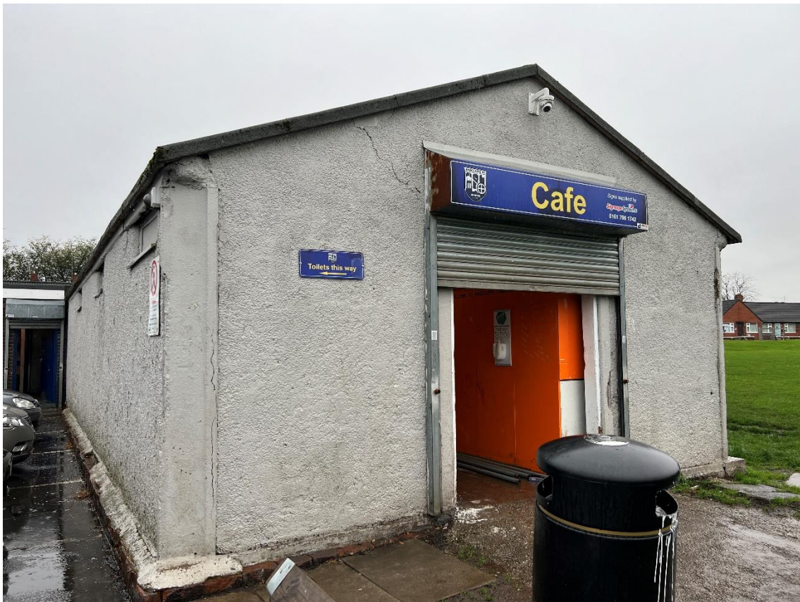
Photograph 1: The east and south aspect of the building (pre-cast concrete structure).
