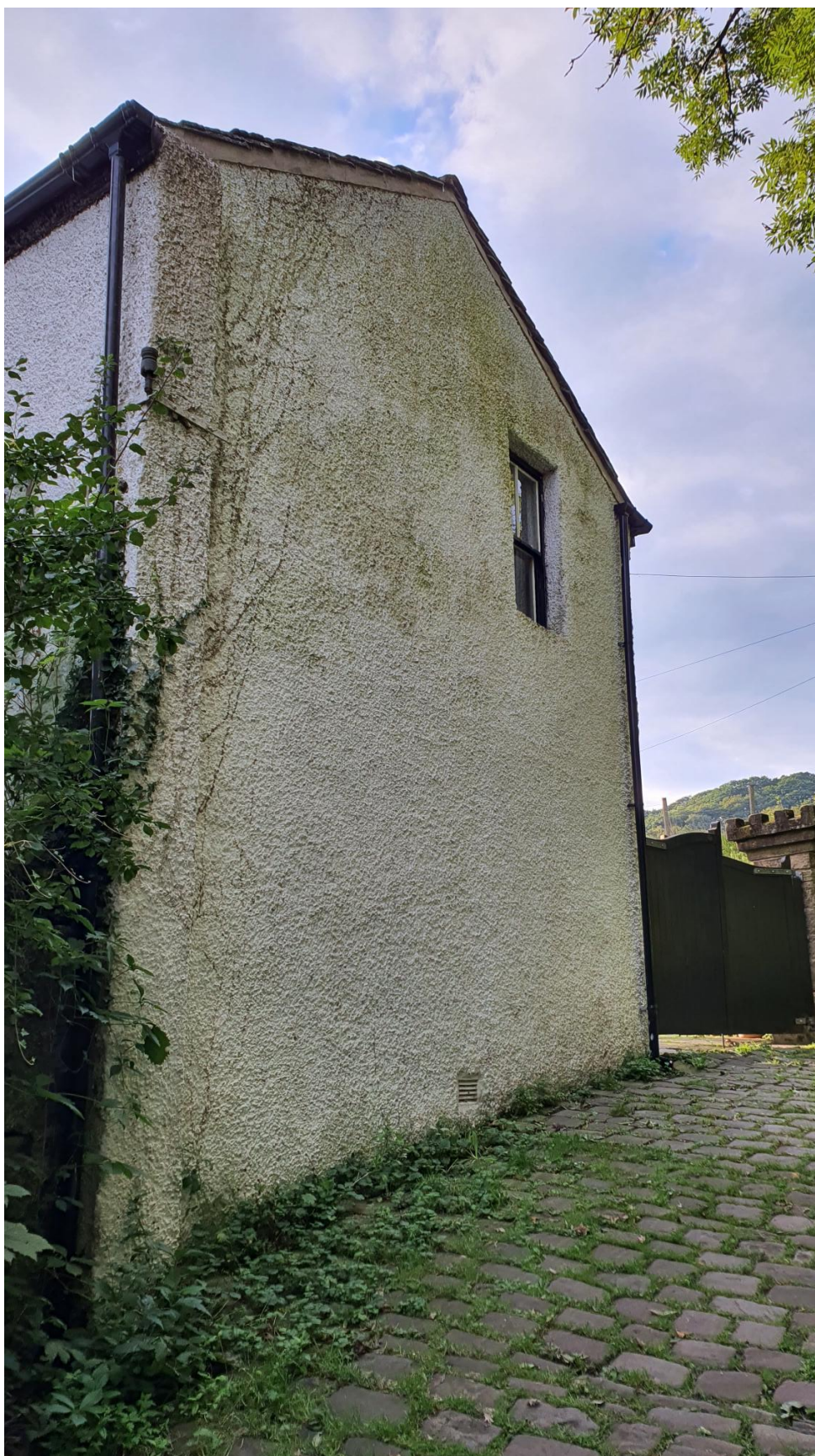
View 1 of side of property (looking at existing window to first floor Bedroom)
