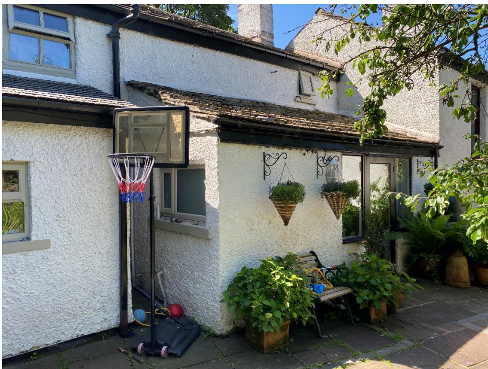
View of rear of property (looking at exterior of existing Bathroom & rear Hall)
