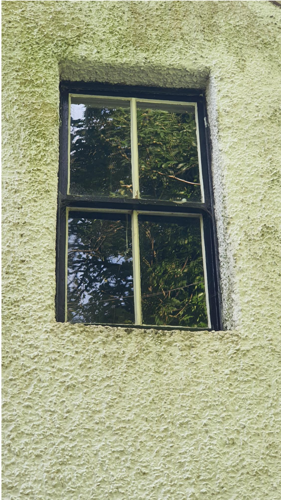
View 2 of side of property (looking at existing window to first floor Bedroom)
