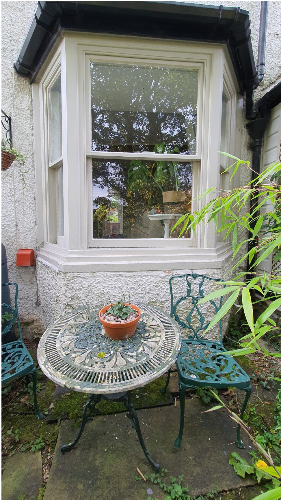
View of front of property (looking at existing bay window to Lounge)
