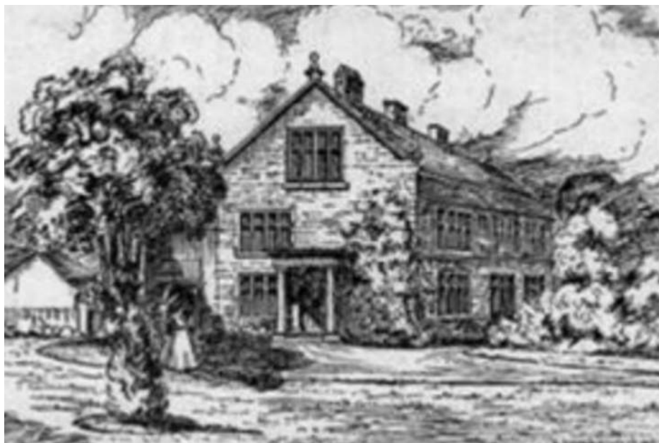
Figure 2 Image showing the original structure to the West; now demolished.
