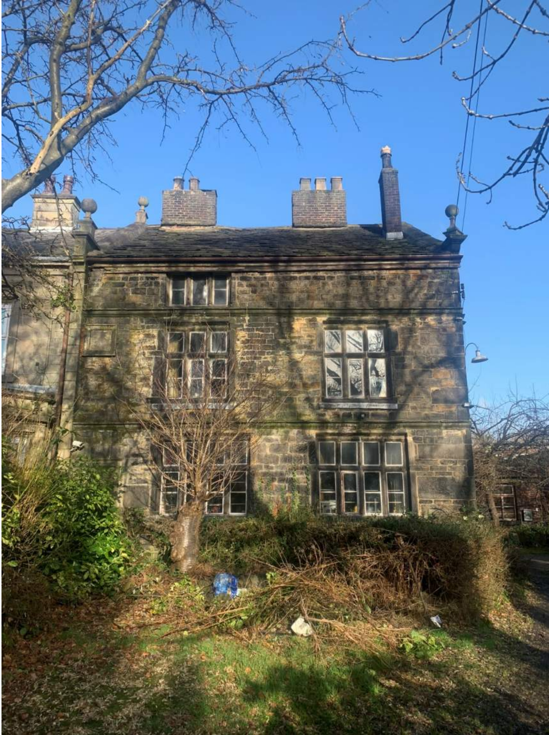
Figure 4 Full view of South Elevation
