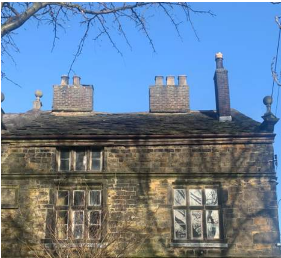
Figure 5 Image showing the three chimneys
