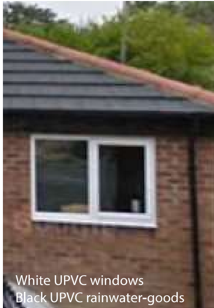
Slate roof to existing house slate look concrete tiles to extension
