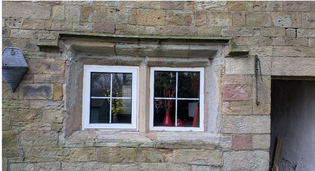
Figure 16: Left-hand side double recessed mullioned window
