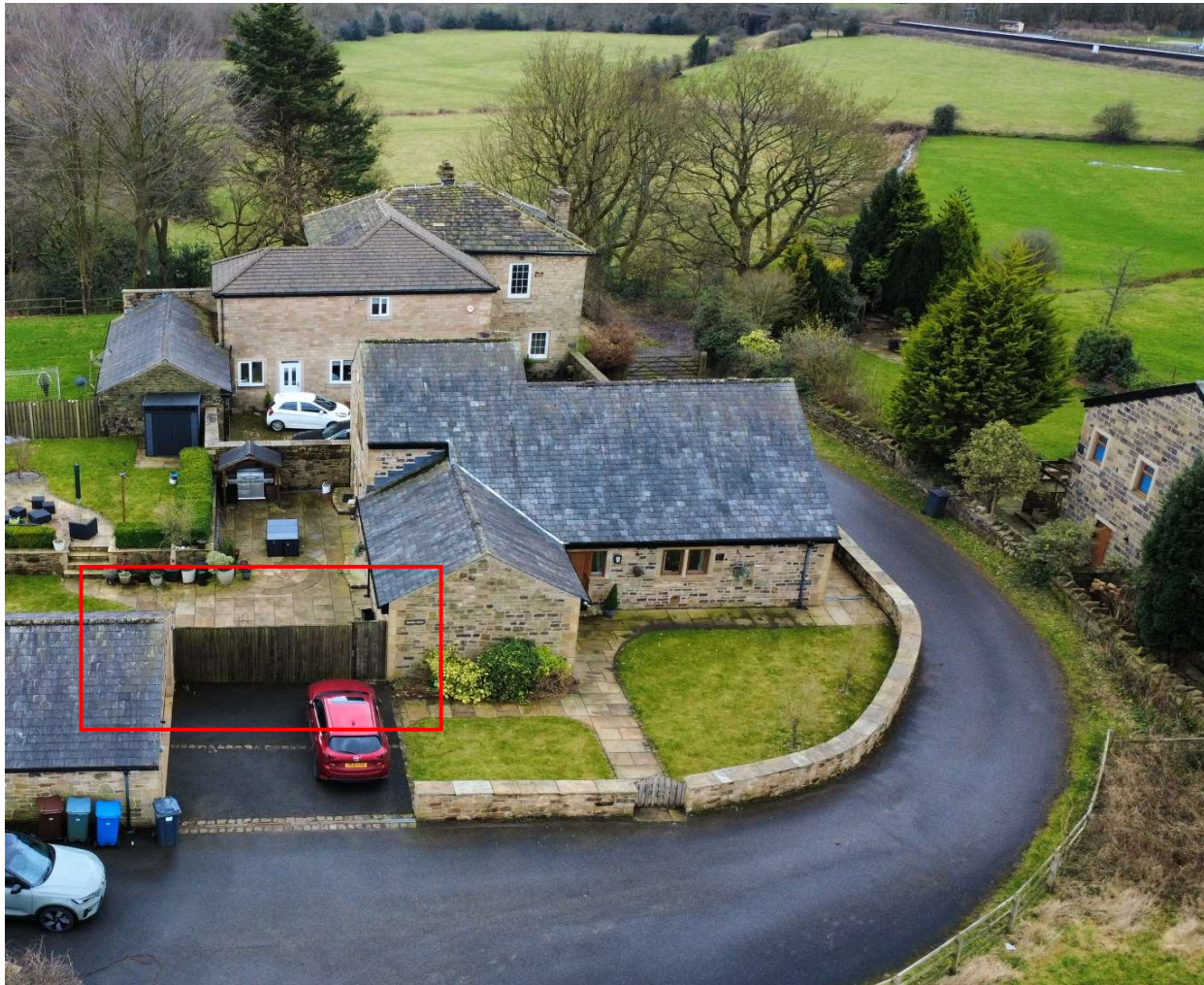
Figure 5: View looking directly over where proposed extension will be approximately erected (red outline)
