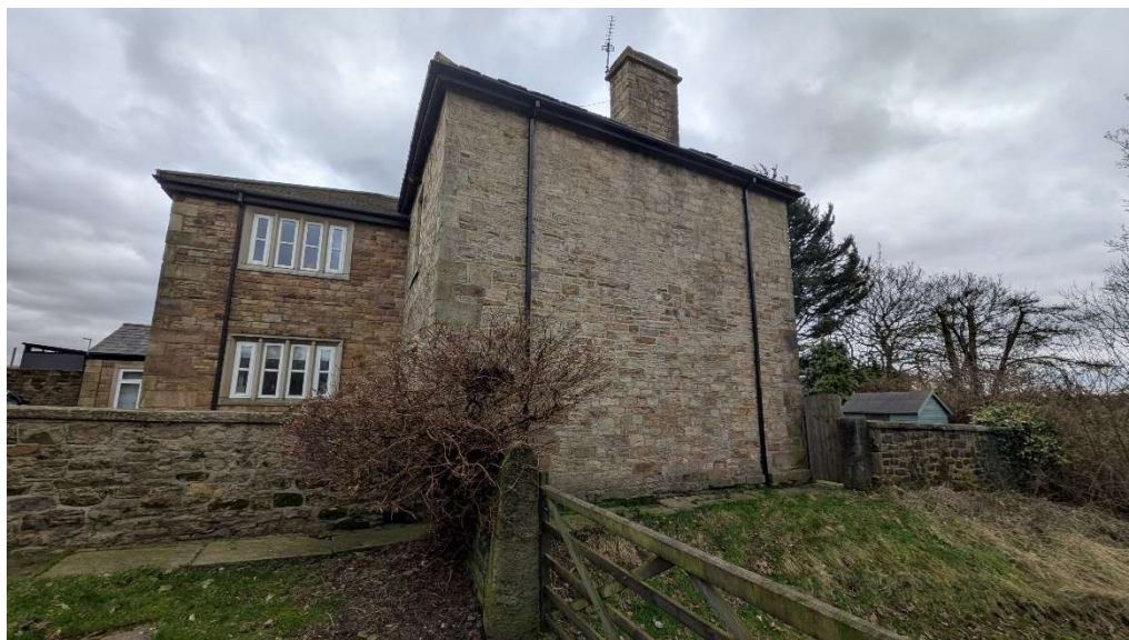
Figure 11: West elevation Touch Road Farmhouse
