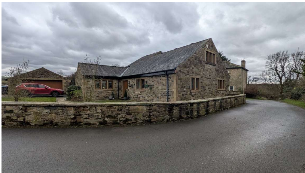
Figure 8: West elevation of Burrs View and road leading to Touch Road Farmhouse
