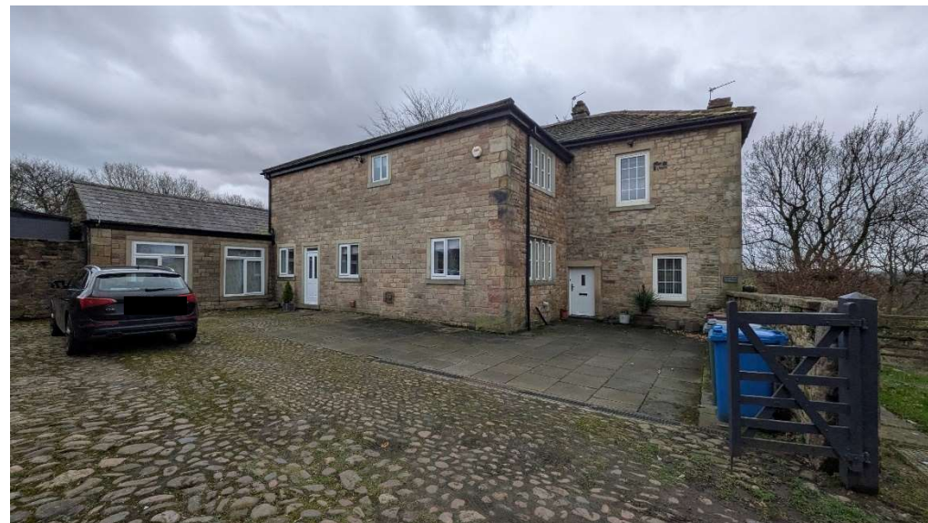
Figure 9: Rear (North) elevation of Touch Road Farmhouse
