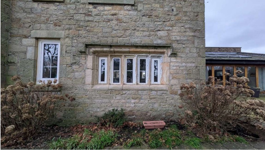
Figure 14: Right-hand side double recessed mullioned window
