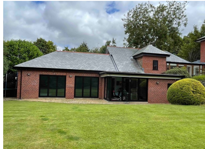
(4) Lower ground building, view from garden
