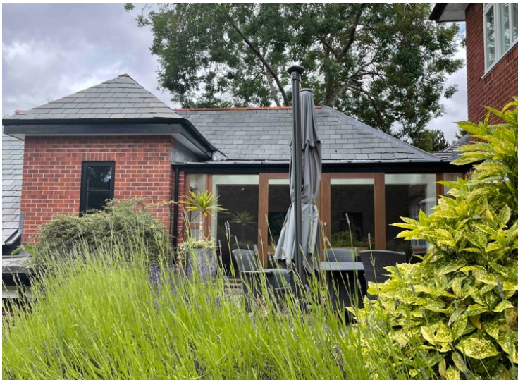
(5) Rear View – Main house side view from terrace
