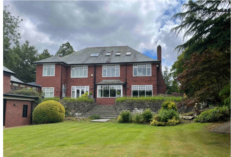
(2) Rear view of main house from garden
