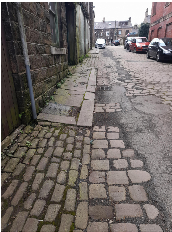
View 1 existing pavement
