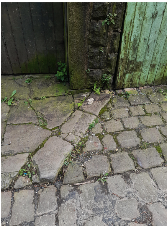
View 3 detail existing pavement
