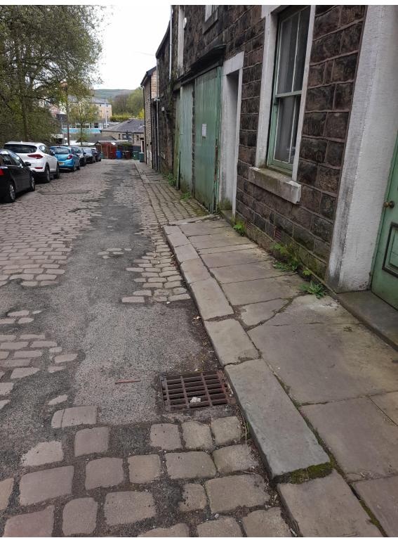
View 2 existing pavement
