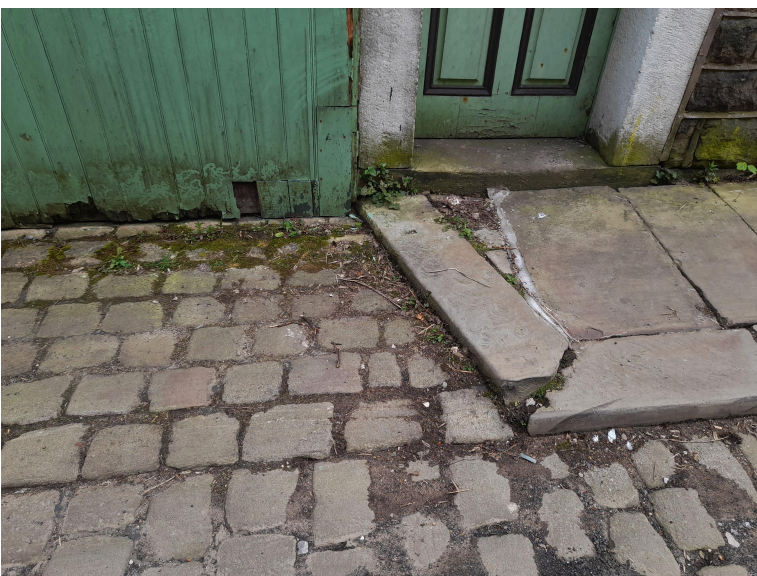
View 4 detail existing pavement
