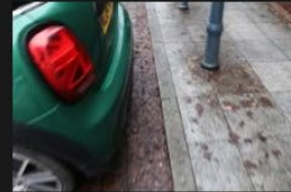
9A-9B – Access Road – Kerb and Footpath - 18-01-2026 (41)
