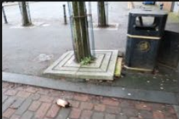
9A-9B – Access Road – Kerb and Footpath - 18-01-2026 (44)
