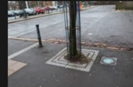
9A-9B – Access Road – Kerb and Footpath - 18-01-2026 (48)
