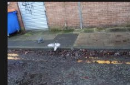
9A-9B – Access Road – Kerb and Footpath - 18-01-2026 (54)
