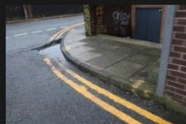
9A-9B – Access Road – Kerb and Footpath - 18-01-2026 (83)
