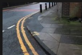
9A-9B – Access Road – Kerb and Footpath - 18-01-2026 (89)
