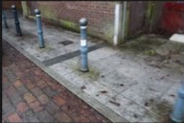
9A-9B – Access Road – Kerb and Footpath - 18-01-2026 (38)
