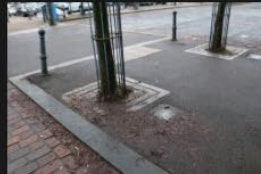
9A-9B – Access Road – Kerb and Footpath - 18-01-2026 (46)
