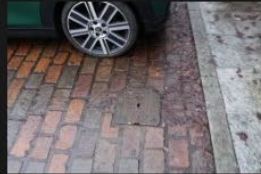
9A-9B – Access Road – Kerb and Footpath - 18-01-2026 (40)
