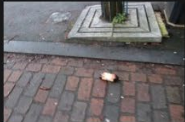
9A-9B – Access Road – Kerb and Footpath - 18-01-2026 (45)
