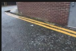
9A-9B – Access Road – Kerb and Footpath - 18-01-2026 (81)
