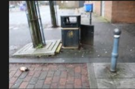
9A-9B – Access Road – Kerb and Footpath - 18-01-2026 (43)
