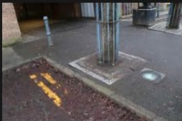
9A-9B – Access Road – Kerb and Footpath - 18-01-2026 (50)
