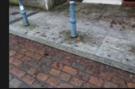
9A-9B – Access Road – Kerb and Footpath - 18-01-2026 (37)
