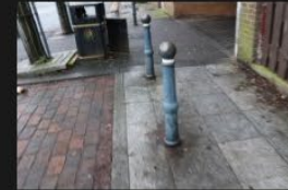
9A-9B – Access Road – Kerb and Footpath - 18-01-2026 (42)
