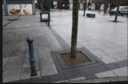
9A-9B – Access Road – Kerb and Footpath - 18-01-2026 (33)
