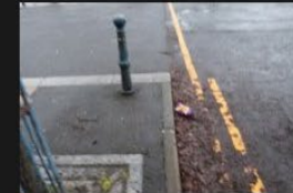
9A-9B – Access Road – Kerb and Footpath - 18-01-2026 (49)
