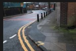
9A-9B – Access Road – Kerb and Footpath - 18-01-2026 (90)
