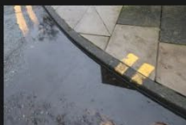
9A-9B – Access Road – Kerb and Footpath - 18-01-2026 (87)
