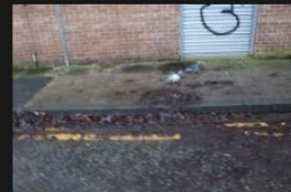
9A-9B – Access Road – Kerb and Footpath - 18-01-2026 (53)
