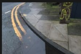
9A-9B – Access Road – Kerb and Footpath - 18-01-2026 (88)
