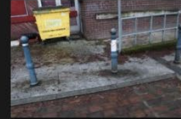
9A-9B – Access Road – Kerb and Footpath - 18-01-2026 (36)
