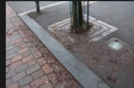
9A-9B – Access Road – Kerb and Footpath - 18-01-2026 (47)
