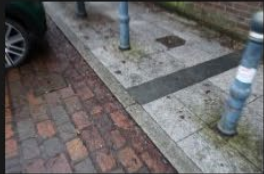
9A-9B – Access Road – Kerb and Footpath - 18-01-2026 (39)
