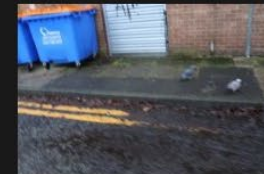
9A-9B – Access Road – Kerb and Footpath - 18-01-2026 (55)
