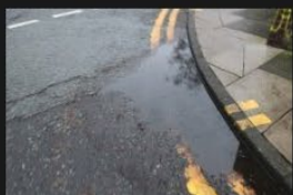
9A-9B – Access Road – Kerb and Footpath - 18-01-2026 (86)
