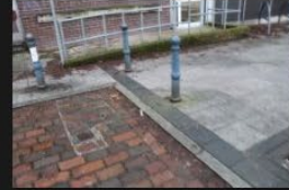
9A-9B – Access Road – Kerb and Footpath - 18-01-2026 (35)
