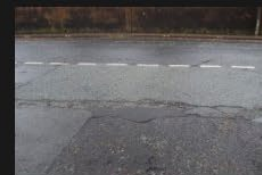
9A-9B – Access Road – Kerb and Footpath - 18-01-2026 (85)
