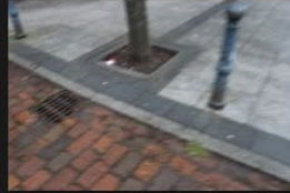
9A-9B – Access Road – Kerb and Footpath - 18-01-2026 (34)
