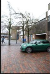
9A-9B – Access Road – Kerb and Footpath - 18-01-2026 (1)
