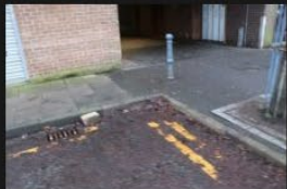
9A-9B – Access Road – Kerb and Footpath - 18-01-2026 (51)
