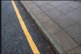
8A-8B – Access Road – Kerbs and Footpath - 18-01-2026 (13)
