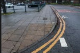
8A-8B – Access Road – Kerbs and Footpath - 18-01-2026 (2)
