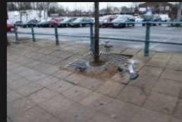
8A-8B – Access Road – Kerbs and Footpath - 18-01-2026 (22)
