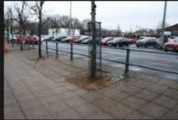
8A-8B – Access Road – Kerbs and Footpath - 18-01-2026 (15)
