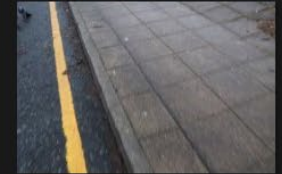
8A-8B – Access Road – Kerbs and Footpath - 18-01-2026 (18)
