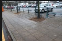
8A-8B – Access Road – Kerbs and Footpath - 18-01-2026 (10)
