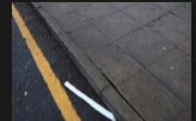
8A-8B – Access Road – Kerbs and Footpath - 18-01-2026 (24)
