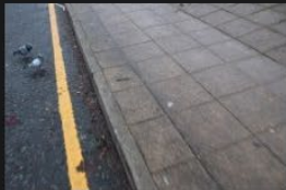
8A-8B – Access Road – Kerbs and Footpath - 18-01-2026 (19)
