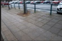
8A-8B – Access Road – Kerbs and Footpath - 18-01-2026 (14)
