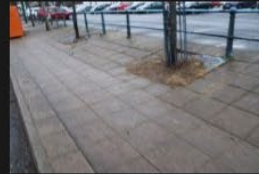
8A-8B – Access Road – Kerbs and Footpath - 18-01-2026 (16)
