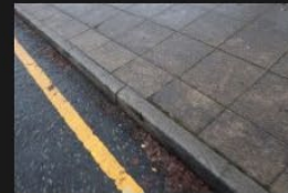
8A-8B – Access Road – Kerbs and Footpath - 18-01-2026 (11)
