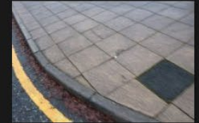
8A-8B – Access Road – Kerbs and Footpath - 18-01-2026 (6)
