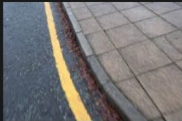
8A-8B – Access Road – Kerbs and Footpath - 18-01-2026 (7)
