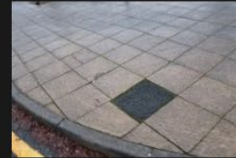
8A-8B – Access Road – Kerbs and Footpath - 18-01-2026 (5)
