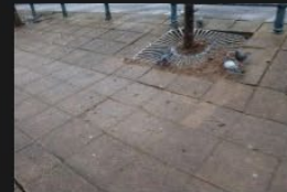
8A-8B – Access Road – Kerbs and Footpath - 18-01-2026 (23)
