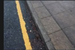
8A-8B – Access Road – Kerbs and Footpath - 18-01-2026 (17)
