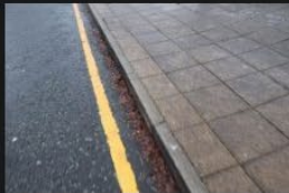
8A-8B – Access Road – Kerbs and Footpath - 18-01-2026 (8)
