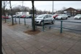
8A-8B – Access Road – Kerbs and Footpath - 18-01-2026 (9)
