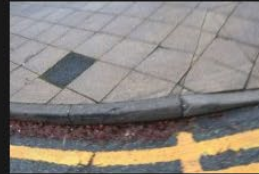
8A-8B – Access Road – Kerbs and Footpath - 18-01-2026 (4)
