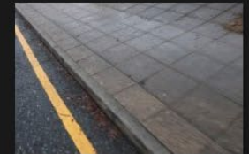
8A-8B – Access Road – Kerbs and Footpath - 18-01-2026 (12)
