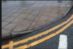
8A-8B – Access Road – Kerbs and Footpath - 18-01-2026 (3)
