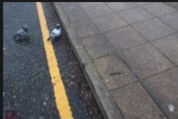
8A-8B – Access Road – Kerbs and Footpath - 18-01-2026 (20)
