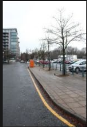
8A-8B – Access Road – Kerbs and Footpath - 18-01-2026 (1)
