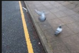
8A-8B – Access Road – Kerbs and Footpath - 18-01-2026 (21)
