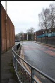
7A-7B - Rectory Lane - Road Surface - 18-01-2026 (79)
