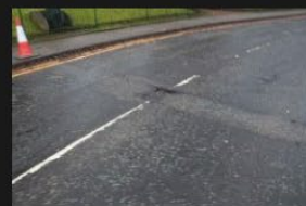
7A-7B - Rectory Lane - Road Surface - 18-01-2026 (12)
