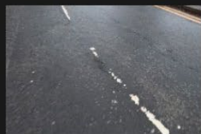
7A-7B - Rectory Lane - Road Surface - 18-01-2026 (7)
