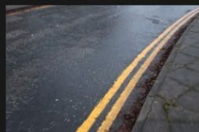
7A-7B - Rectory Lane - Road Surface - 18-01-2026 (19)
