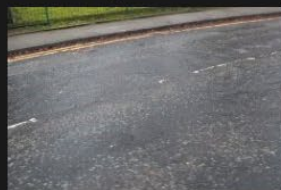
7A-7B - Rectory Lane - Road Surface - 18-01-2026 (15)
