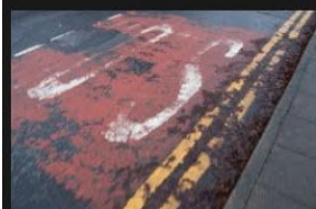
7A-7B - Rectory Lane - Road Surface - 18-01-2026 (43)
