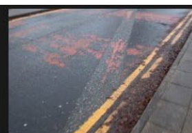
7A-7B - Rectory Lane - Road Surface - 18-01-2026 (29)
