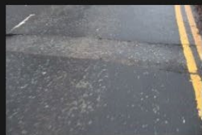
7A-7B - Rectory Lane - Road Surface - 18-01-2026 (13)
