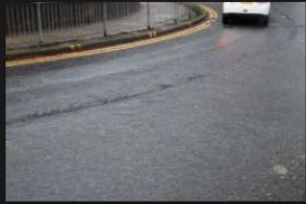
7A-7B - Rectory Lane - Road Surface - 18-01-2026 (73)
