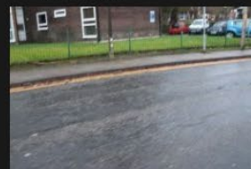
7A-7B - Rectory Lane - Road Surface - 18-01-2026 (24)
