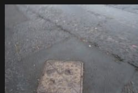
7A-7B - Rectory Lane - Road Surface - 18-01-2026 (5)
