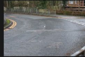
7A-7B - Rectory Lane - Road Surface - 18-01-2026 (77)
