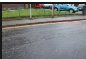
7A-7B - Rectory Lane - Road Surface - 18-01-2026 (26)
