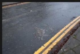
7A-7B - Rectory Lane - Road Surface - 18-01-2026 (21)
