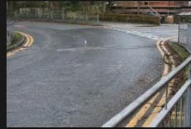
7A-7B - Rectory Lane - Road Surface - 18-01-2026 (76)
