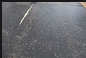
7A-7B - Rectory Lane - Road Surface - 18-01-2026 (10)
