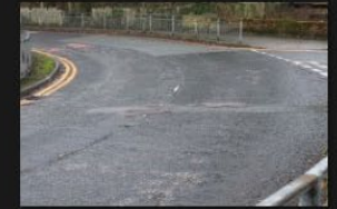
7A-7B - Rectory Lane - Road Surface - 18-01-2026 (78)
