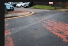
7A-7B - Rectory Lane - Road Surface - 18-01-2026 (36)
