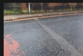
7A-7B - Rectory Lane - Road Surface - 18-01-2026 (47)
