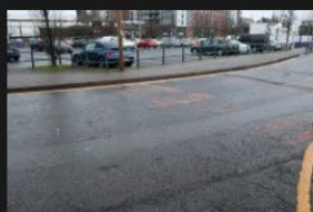
7A-7B - Rectory Lane - Road Surface - 18-01-2026 (2)
