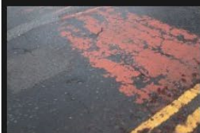
7A-7B - Rectory Lane - Road Surface - 18-01-2026 (37)
