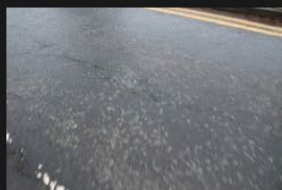
7A-7B - Rectory Lane - Road Surface - 18-01-2026 (8)
