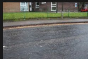
7A-7B - Rectory Lane - Road Surface - 18-01-2026 (23)
