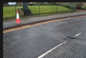
7A-7B - Rectory Lane - Road Surface - 18-01-2026 (11)
