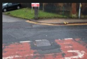
7A-7B - Rectory Lane - Road Surface - 18-01-2026 (45)
