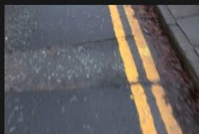
7A-7B - Rectory Lane - Road Surface - 18-01-2026 (14)
