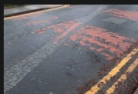
7A-7B - Rectory Lane - Road Surface - 18-01-2026 (33)
