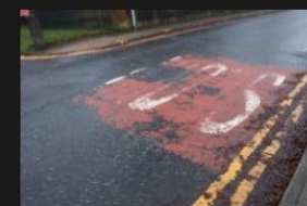
7A-7B - Rectory Lane - Road Surface - 18-01-2026 (42)
