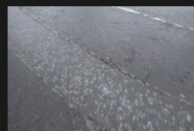
7A-7B - Rectory Lane - Road Surface - 18-01-2026 (6)
