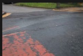
7A-7B - Rectory Lane - Road Surface - 18-01-2026 (39)
