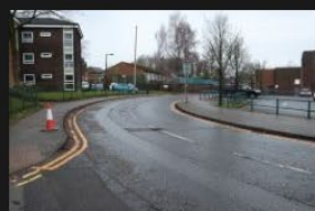
7A-7B - Rectory Lane - Road Surface - 18-01-2026 (1)
