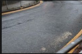
7A-7B - Rectory Lane - Road Surface - 18-01-2026 (74)
