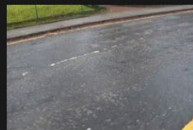
7A-7B - Rectory Lane - Road Surface - 18-01-2026 (17)
