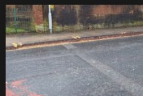
7A-7B - Rectory Lane - Road Surface - 18-01-2026 (46)
