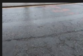
7A-7B - Rectory Lane - Road Surface - 18-01-2026 (3)
