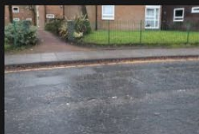
7A-7B - Rectory Lane - Road Surface - 18-01-2026 (20)
