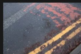
7A-7B - Rectory Lane - Road Surface - 18-01-2026 (34)
