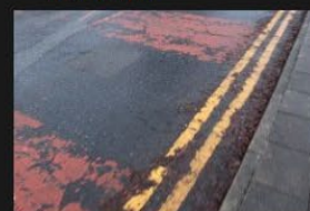
7A-7B - Rectory Lane - Road Surface - 18-01-2026 (35)
