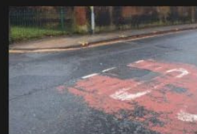
7A-7B - Rectory Lane - Road Surface - 18-01-2026 (41)
