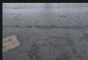
7A-7B - Rectory Lane - Road Surface - 18-01-2026 (4)
