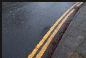
7A-7B - Rectory Lane - Road Surface - 18-01-2026 (22)
