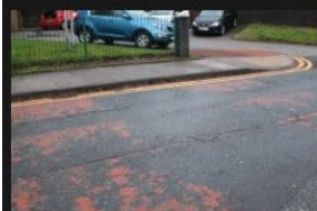
7A-7B - Rectory Lane - Road Surface - 18-01-2026 (31)
