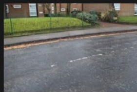
7A-7B - Rectory Lane - Road Surface - 18-01-2026 (16)
