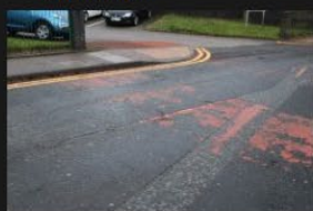
7A-7B - Rectory Lane - Road Surface - 18-01-2026 (32)
