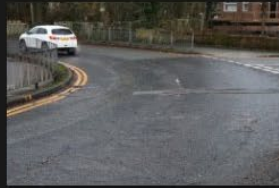
7A-7B - Rectory Lane - Road Surface - 18-01-2026 (75)
