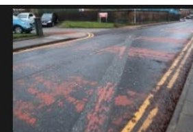
7A-7B - Rectory Lane - Road Surface - 18-01-2026 (30)
