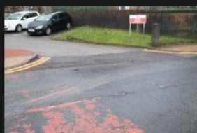
7A-7B - Rectory Lane - Road Surface - 18-01-2026 (38)
