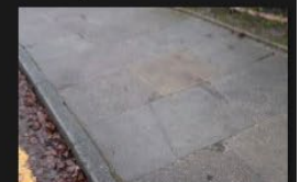
6A-6B – Rectory Lane – Kerbs and Footpath - 18-01-2026 (72)
