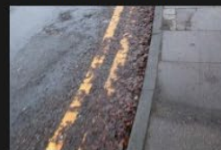
6A-6B - Rectory Lane - Kerbs and Footpath - 18-01-2026 (83)
