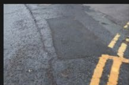
6A-6B - Rectory Lane - Kerbs and Footpath - 18-01-2026 (91)
