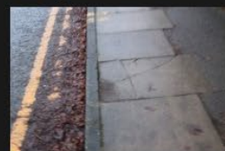
6A-6B – Rectory Lane – Kerbs and Footpath - 18-01-2026 (41)
