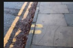
6A-6B – Rectory Lane – Kerbs and Footpath - 18-01-2026 (48)
