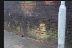
6A-6B – Rectory Lane – Kerbs and Footpath - 18-01-2026 (16)
