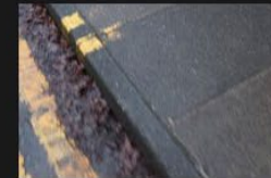
6A-6B – Rectory Lane – Kerbs and Footpath - 18-01-2026 (17)
