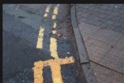
6A-6B - Rectory Lane - Kerbs and Footpath - 18-01-2026 (92)
