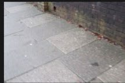
6A-6B – Rectory Lane – Kerbs and Footpath - 18-01-2026 (20)
