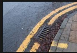
6A-6B – Rectory Lane – Kerbs and Footpath - 18-01-2026 (51)
