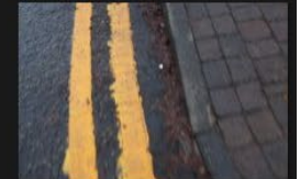
6A-6B – Rectory Lane – Kerbs and Footpath - 18-01-2026 (60)
