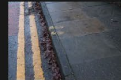
6A-6B – Rectory Lane – Kerbs and Footpath - 18-01-2026 (23)
