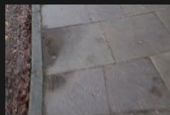
6A-6B - Rectory Lane - Kerbs and Footpath - 18-01-2026 (82)
