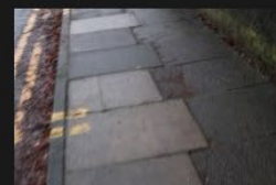
6A-6B – Rectory Lane – Kerbs and Footpath - 18-01-2026 (42)
