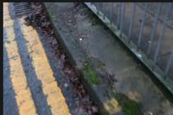
6A-6B – Rectory Lane – Kerbs and Footpath - 18-01-2026 (13)
