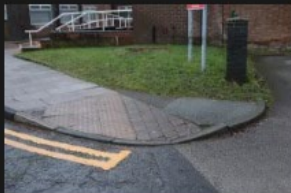
6A-6B – Rectory Lane – Kerbs and Footpath - 18-01-2026 (98)
