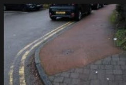
6A-6B - Rectory Lane - Kerbs and Footpath - 18-01-2026 (94)
