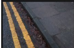
6A-6B – Rectory Lane – Kerbs and Footpath - 18-01-2026 (67)
