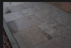
6A-6B - Rectory Lane - Kerbs and Footpath - 18-01-2026 (77)
