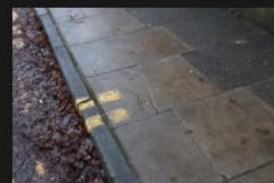
6A-6B – Rectory Lane – Kerbs and Footpath - 18-01-2026 (35)
