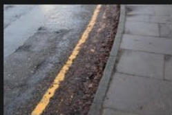
6A-6B - Rectory Lane - Kerbs and Footpath - 18-01-2026 (80)
