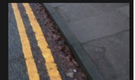
6A-6B – Rectory Lane – Kerbs and Footpath - 18-01-2026 (66)
