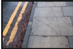
6A-6B – Rectory Lane – Kerbs and Footpath - 18-01-2026 (49)
