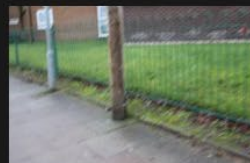
6A-6B – Rectory Lane – Kerbs and Footpath - 18-01-2026 (63)
