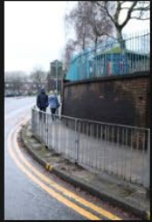
6A-6B – Rectory Lane – Kerbs and Footpath - 18-01-2026 (1)
