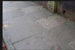
6A-6B – Rectory Lane – Kerbs and Footpath - 18-01-2026 (21)
