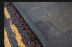
6A-6B – Rectory Lane – Kerbs and Footpath - 18-01-2026 (71)
