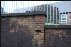
6A-6B – Rectory Lane – Kerbs and Footpath - 18-01-2026 (7)
