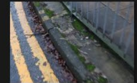
6A-6B – Rectory Lane – Kerbs and Footpath - 18-01-2026 (12)
