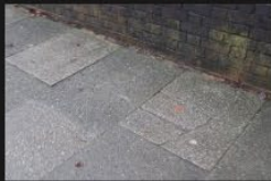
6A-6B – Rectory Lane – Kerbs and Footpath - 18-01-2026 (19)
