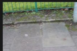
6A-6B – Rectory Lane – Kerbs and Footpath - 18-01-2026 (69)
