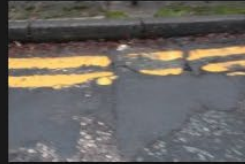
6A-6B – Rectory Lane – Kerbs and Footpath - 18-01-2026 (3)
