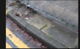
6A-6B – Rectory Lane – Kerbs and Footpath - 18-01-2026 (6)
