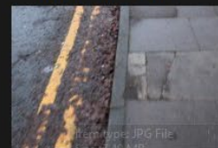
6A-6B - Rectory Lane - Kerbs and Footpath - 18-01-2026 (84)
