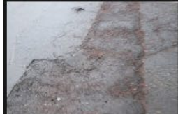
6A-6B – Rectory Lane – Kerbs and Footpath - 18-01-2026 (55)
