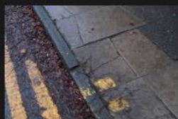
6A-6B – Rectory Lane – Kerbs and Footpath - 18-01-2026 (38)
