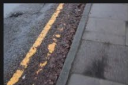
6A-6B - Rectory Lane - Kerbs and Footpath - 18-01-2026 (79)
