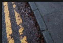
6A-6B - Rectory Lane - Kerbs and Footpath - 18-01-2026 (76)
