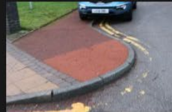
6A-6B – Rectory Lane – Kerbs and Footpath - 18-01-2026 (57)
