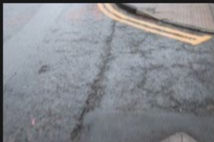
6A-6B – Rectory Lane – Kerbs and Footpath - 18-01-2026 (97)
