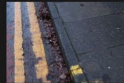
6A-6B – Rectory Lane – Kerbs and Footpath - 18-01-2026 (22)
