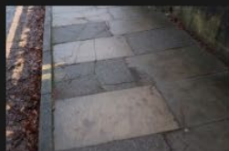
6A-6B – Rectory Lane – Kerbs and Footpath - 18-01-2026 (44)
