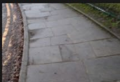
6A-6B - Rectory Lane - Kerbs and Footpath - 18-01-2026 (81)
