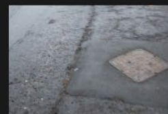
6A-6B - Rectory Lane - Kerbs and Footpath - 18-01-2026 (96)
