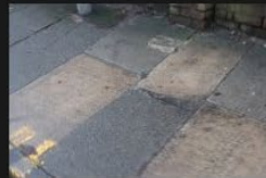
6A-6B – Rectory Lane – Kerbs and Footpath - 18-01-2026 (15)
