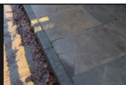
6A-6B – Rectory Lane – Kerbs and Footpath - 18-01-2026 (27)
