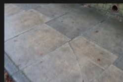
6A-6B – Rectory Lane – Kerbs and Footpath - 18-01-2026 (34)
