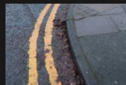
6A-6B - Rectory Lane - Kerbs and Footpath - 18-01-2026 (89)
