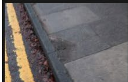
6A-6B – Rectory Lane – Kerbs and Footpath - 18-01-2026 (61)
