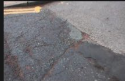
6A-6B – Rectory Lane – Kerbs and Footpath - 18-01-2026 (56)
