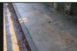
6A-6B – Rectory Lane – Kerbs and Footpath - 18-01-2026 (29)
