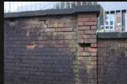
6A-6B – Rectory Lane – Kerbs and Footpath - 18-01-2026 (8)
