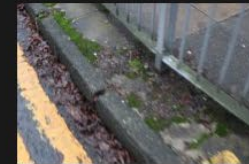
6A-6B – Rectory Lane – Kerbs and Footpath - 18-01-2026 (11)
