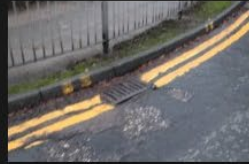
6A-6B – Rectory Lane – Kerbs and Footpath - 18-01-2026 (2)
