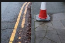
6A-6B - Rectory Lane - Kerbs and Footpath - 18-01-2026 (86)
