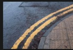
6A-6B – Rectory Lane – Kerbs and Footpath - 18-01-2026 (52)
