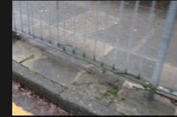
6A-6B – Rectory Lane – Kerbs and Footpath - 18-01-2026 (5)
