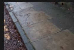
6A-6B – Rectory Lane – Kerbs and Footpath - 18-01-2026 (36)
