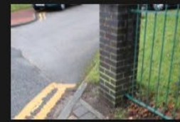
6A-6B – Rectory Lane – Kerbs and Footpath - 18-01-2026 (53)
