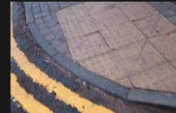
6A-6B – Rectory Lane – Kerbs and Footpath - 18-01-2026 (59)
