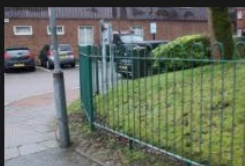
6A-6B - Rectory Lane - Kerbs and Footpath - 18-01-2026 (87)
