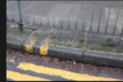
6A-6B – Rectory Lane – Kerbs and Footpath - 18-01-2026 (4)
