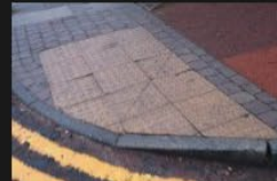
6A-6B – Rectory Lane – Kerbs and Footpath - 18-01-2026 (58)
