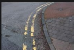
6A-6B - Rectory Lane - Kerbs and Footpath - 18-01-2026 (93)
