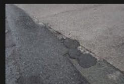
6A-6B - Rectory Lane - Kerbs and Footpath - 18-01-2026 (95)
