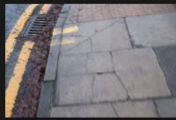
6A-6B – Rectory Lane – Kerbs and Footpath - 18-01-2026 (50)
