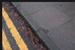
6A-6B – Rectory Lane – Kerbs and Footpath - 18-01-2026 (68)
