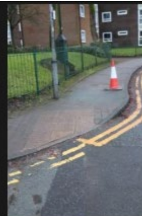
6A-6B – Rectory Lane – Kerbs and Footpath - 18-01-2026 (99)
