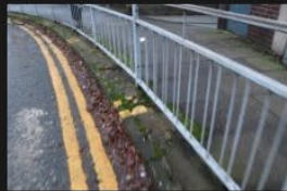
5A-5B – Rectory Lane – Kerbs and Footpath - 18-01-2026 (85)
