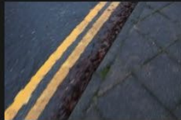
5A-5B – Rectory Lane – Kerbs and Footpath - 18-01-2026 (20)
