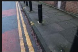
5A-5B – Rectory Lane – Kerbs and Footpath - 18-01-2026 (73)
