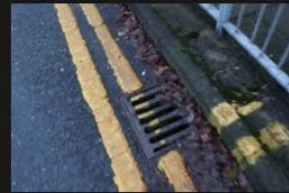
5A-5B – Rectory Lane – Kerbs and Footpath - 18-01-2026 (82)
