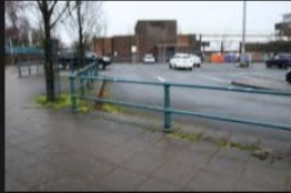
5A-5B – Rectory Lane – Kerbs and Footpath - 18-01-2026 (13)
