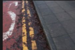
5A-5B – Rectory Lane – Kerbs and Footpath - 18-01-2026 (45)
