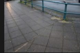
5A-5B – Rectory Lane – Kerbs and Footpath - 18-01-2026 (6)
