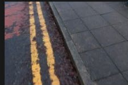
5A-5B – Rectory Lane – Kerbs and Footpath - 18-01-2026 (39)
