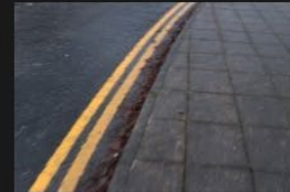
5A-5B – Rectory Lane – Kerbs and Footpath - 18-01-2026 (11)
