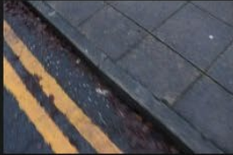
5A-5B – Rectory Lane – Kerbs and Footpath - 18-01-2026 (31)
