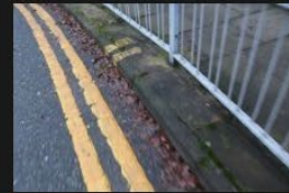
5A-5B – Rectory Lane – Kerbs and Footpath - 18-01-2026 (83)
