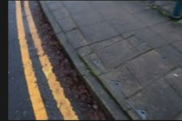
5A-5B – Rectory Lane – Kerbs and Footpath - 18-01-2026 (28)
