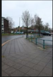
5A-5B – Rectory Lane – Kerbs and Footpath - 18-01-2026 (1)
