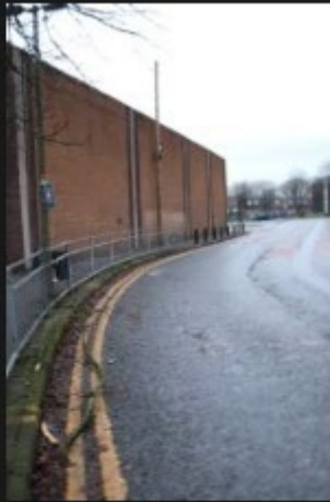
☁ 5A-5B – Rectory Lane – Kerbs and Footpath - 18-01-2026 (98)
