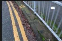
5A-5B – Rectory Lane – Kerbs and Footpath - 18-01-2026 (87)
