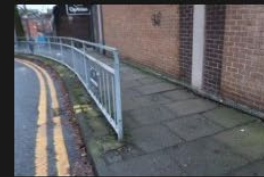
5A-5B – Rectory Lane – Kerbs and Footpath - 18-01-2026 (78)
