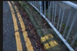
5A-5B – Rectory Lane – Kerbs and Footpath - 18-01-2026 (88)
