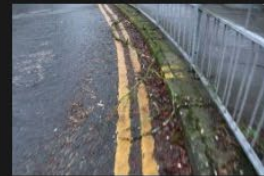
5A-5B – Rectory Lane – Kerbs and Footpath - 18-01-2026 (89)
