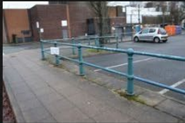
5A-5B – Rectory Lane – Kerbs and Footpath - 18-01-2026 (43)
