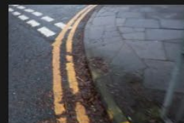
5A-5B – Rectory Lane – Kerbs and Footpath - 18-01-2026 (95)
