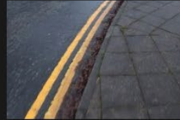
5A-5B – Rectory Lane – Kerbs and Footpath - 18-01-2026 (16)
