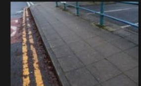
5A-5B – Rectory Lane – Kerbs and Footpath - 18-01-2026 (42)
