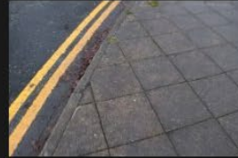
5A-5B – Rectory Lane – Kerbs and Footpath - 18-01-2026 (4)
