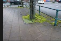
5A-5B – Rectory Lane – Kerbs and Footpath - 18-01-2026 (17)
