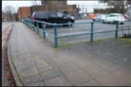
5A-5B – Rectory Lane – Kerbs and Footpath - 18-01-2026 (25)
