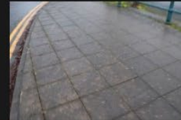
5A-5B – Rectory Lane – Kerbs and Footpath - 18-01-2026 (12)
