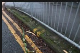
5A-5B – Rectory Lane – Kerbs and Footpath - 18-01-2026 (92)
