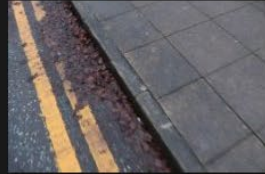
5A-5B – Rectory Lane – Kerbs and Footpath - 18-01-2026 (32)
