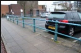
5A-5B – Rectory Lane – Kerbs and Footpath - 18-01-2026 (37)
