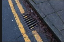
5A-5B – Rectory Lane – Kerbs and Footpath - 18-01-2026 (26)
