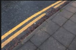
5A-5B – Rectory Lane – Kerbs and Footpath - 18-01-2026 (7)
