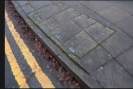
5A-5B – Rectory Lane – Kerbs and Footpath - 18-01-2026 (27)
