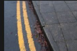
5A-5B – Rectory Lane – Kerbs and Footpath - 18-01-2026 (24)
