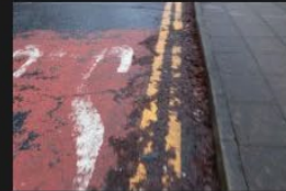
5A-5B – Rectory Lane – Kerbs and Footpath - 18-01-2026 (46)
