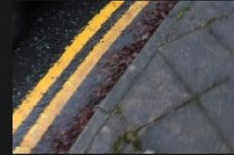
5A-5B – Rectory Lane – Kerbs and Footpath - 18-01-2026 (18)
