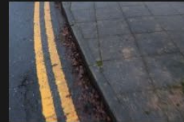
5A-5B – Rectory Lane – Kerbs and Footpath - 18-01-2026 (23)
