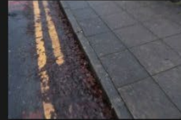
5A-5B – Rectory Lane – Kerbs and Footpath - 18-01-2026 (34)
