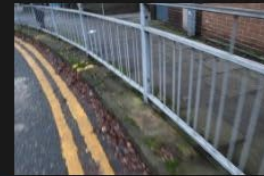
5A-5B – Rectory Lane – Kerbs and Footpath - 18-01-2026 (84)
