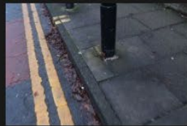
5A-5B – Rectory Lane – Kerbs and Footpath - 18-01-2026 (75)
