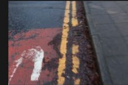
5A-5B – Rectory Lane – Kerbs and Footpath - 18-01-2026 (47)
