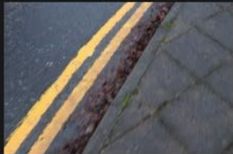
5A-5B – Rectory Lane – Kerbs and Footpath - 18-01-2026 (19)
