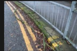
5A-5B – Rectory Lane – Kerbs and Footpath - 18-01-2026 (90)
