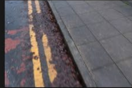
5A-5B – Rectory Lane – Kerbs and Footpath - 18-01-2026 (33)
