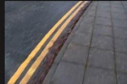
5A-5B – Rectory Lane – Kerbs and Footpath - 18-01-2026 (10)
