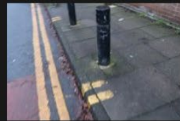
5A-5B – Rectory Lane – Kerbs and Footpath - 18-01-2026 (76)
