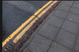
5A-5B – Rectory Lane – Kerbs and Footpath - 18-01-2026 (9)
