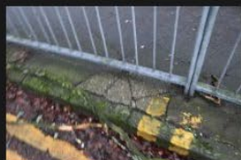
5A-5B – Rectory Lane – Kerbs and Footpath - 18-01-2026 (91)
