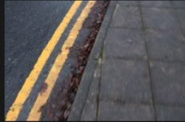
5A-5B – Rectory Lane – Kerbs and Footpath - 18-01-2026 (14)
