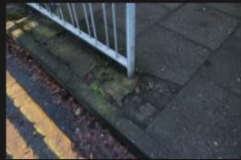
5A-5B – Rectory Lane – Kerbs and Footpath - 18-01-2026 (80)
