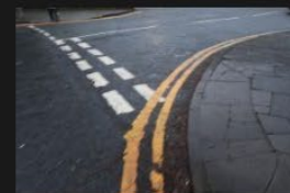
5A-5B – Rectory Lane – Kerbs and Footpath - 18-01-2026 (96)
