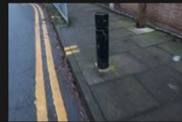
5A-5B – Rectory Lane – Kerbs and Footpath - 18-01-2026 (77)
