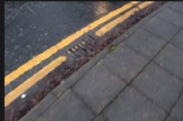
5A-5B – Rectory Lane – Kerbs and Footpath - 18-01-2026 (8)
