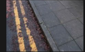
5A-5B – Rectory Lane – Kerbs and Footpath - 18-01-2026 (36)
