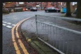
5A-5B – Rectory Lane – Kerbs and Footpath - 18-01-2026 (93)
