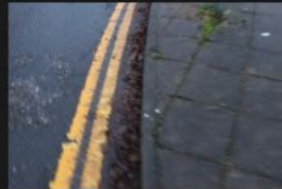
5A-5B – Rectory Lane – Kerbs and Footpath - 18-01-2026 (21)
