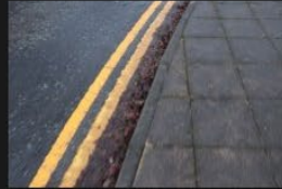
5A-5B – Rectory Lane – Kerbs and Footpath - 18-01-2026 (15)
