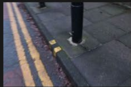
5A-5B – Rectory Lane – Kerbs and Footpath - 18-01-2026 (74)
