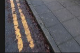
5A-5B – Rectory Lane – Kerbs and Footpath - 18-01-2026 (35)
