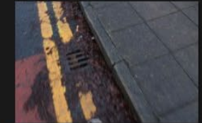
5A-5B – Rectory Lane – Kerbs and Footpath - 18-01-2026 (48)
