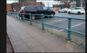
5A-5B – Rectory Lane – Kerbs and Footpath - 18-01-2026 (30)
