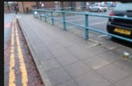
5A-5B – Rectory Lane – Kerbs and Footpath - 18-01-2026 (38)
