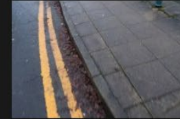
5A-5B – Rectory Lane – Kerbs and Footpath - 18-01-2026 (29)
