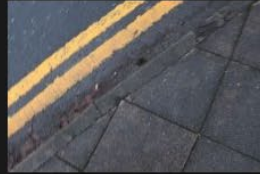
5A-5B – Rectory Lane – Kerbs and Footpath - 18-01-2026 (3)
