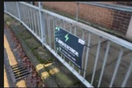
5A-5B – Rectory Lane – Kerbs and Footpath - 18-01-2026 (81)
