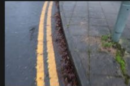
5A-5B – Rectory Lane – Kerbs and Footpath - 18-01-2026 (22)
