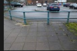
5A-5B – Rectory Lane – Kerbs and Footpath - 18-01-2026 (5)
