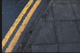
5A-5B – Rectory Lane – Kerbs and Footpath - 18-01-2026 (2)
