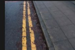
5A-5B – Rectory Lane – Kerbs and Footpath - 18-01-2026 (41)
