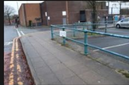
5A-5B – Rectory Lane – Kerbs and Footpath - 18-01-2026 (44)
