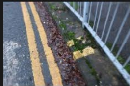
5A-5B – Rectory Lane – Kerbs and Footpath - 18-01-2026 (86)
