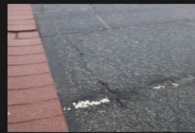
4A-4B - Rectory Lane - Road Surface - 18-01-2026 (28)
