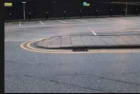
4A-4B - Rectory Lane - Road Surface - 18-01-2026 (37)
