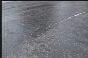
4A-4B - Rectory Lane - Road Surface - 18-01-2026 (109)
