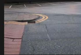
4A-4B - Rectory Lane - Road Surface - 18-01-2026 (29)
