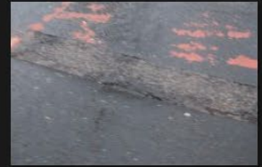
4A-4B - Rectory Lane - Road Surface - 18-01-2026 (102)
