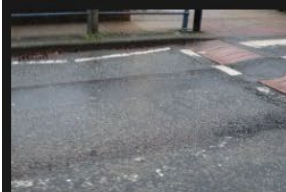
4A-4B - Rectory Lane - Road Surface - 18-01-2026 (61)
