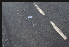
4A-4B - Rectory Lane - Road Surface - 18-01-2026 (57)
