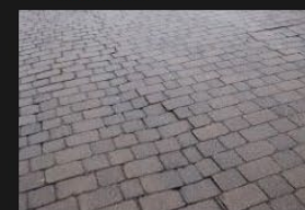
4A-4B – Rectory Lane – Road Surface - 18-01-2026 (12)
