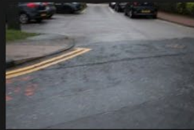
4A-4B - Rectory Lane - Road Surface - 18-01-2026 (106)
