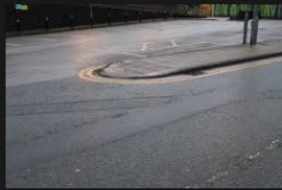
4A-4B - Rectory Lane - Road Surface - 18-01-2026 (32)
