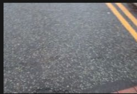
4A-4B - Rectory Lane - Road Surface - 18-01-2026 (27)
