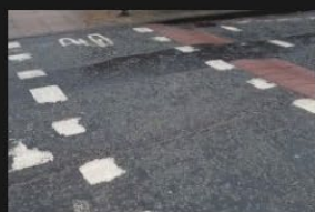
4A-4B - Rectory Lane - Road Surface - 18-01-2026 (68)
