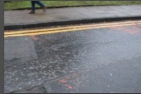
4A-4B - Rectory Lane - Road Surface - 18-01-2026 (100)
