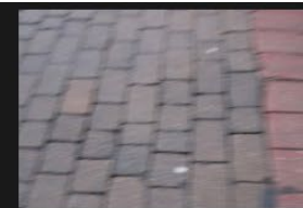
4A-4B – Rectory Lane – Road Surface - 18-01-2026 (6)
