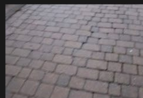
4A-4B – Rectory Lane – Road Surface - 18-01-2026 (16)
