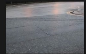
4A-4B - Rectory Lane - Road Surface - 18-01-2026 (30)
