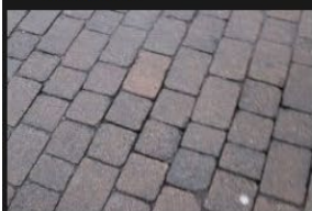
4A-4B – Rectory Lane – Road Surface - 18-01-2026 (7)
