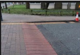
4A-4B – Rectory Lane – Road Surface - 18-01-2026 (2)
