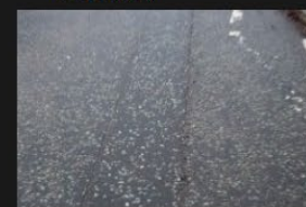
4A-4B - Rectory Lane - Road Surface - 18-01-2026 (59)
