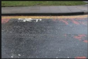
4A-4B - Rectory Lane - Road Surface - 18-01-2026 (104)
