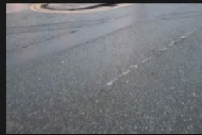
4A-4B - Rectory Lane - Road Surface - 18-01-2026 (31)
