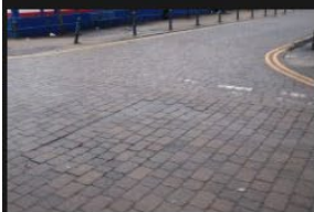
4A-4B – Rectory Lane – Road Surface - 18-01-2026 (13)
