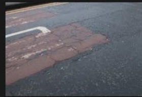
4A-4B - Rectory Lane - Road Surface - 18-01-2026 (46)
