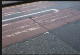
4A-4B - Rectory Lane - Road Surface - 18-01-2026 (45)
