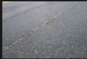
4A-4B - Rectory Lane - Road Surface - 18-01-2026 (33)
