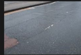
4A-4B - Rectory Lane - Road Surface - 18-01-2026 (47)
