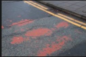
4A-4B - Rectory Lane - Road Surface - 18-01-2026 (97)
