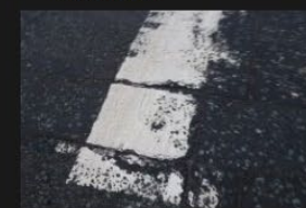
4A-4B - Rectory Lane - Road Surface - 18-01-2026 (66)
