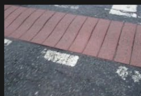
4A-4B - Rectory Lane - Road Surface - 18-01-2026 (63)
