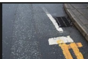
4A-4B - Rectory Lane - Road Surface - 18-01-2026 (50)
