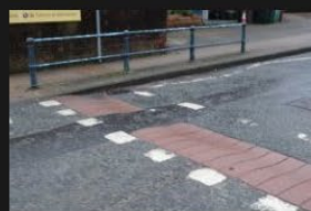
4A-4B - Rectory Lane - Road Surface - 18-01-2026 (69)
