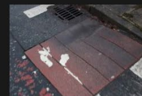
4A-4B - Rectory Lane - Road Surface - 18-01-2026 (72)
