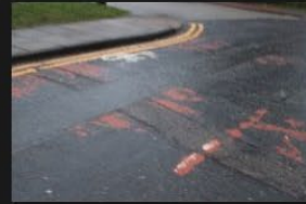
4A-4B - Rectory Lane - Road Surface - 18-01-2026 (101)
