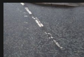
4A-4B - Rectory Lane - Road Surface - 18-01-2026 (58)
