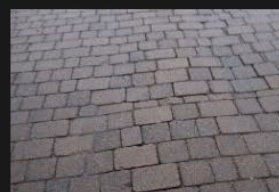
4A-4B – Rectory Lane – Road Surface - 18-01-2026 (10)
