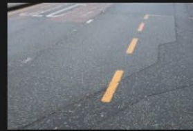
4A-4B - Rectory Lane - Road Surface - 18-01-2026 (40)
