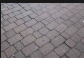
4A-4B – Rectory Lane – Road Surface - 18-01-2026 (8)
