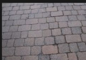
4A-4B – Rectory Lane – Road Surface - 18-01-2026 (9)
