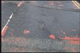
4A-4B - Rectory Lane - Road Surface - 18-01-2026 (98)
