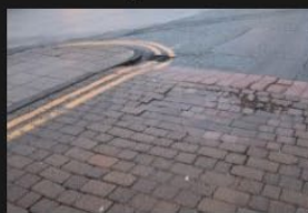
4A-4B – Rectory Lane – Road Surface - 18-01-2026 (21)
