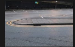
4A-4B - Rectory Lane - Road Surface - 18-01-2026 (36)
