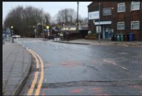
4A-4B - Rectory Lane - Road Surface - 18-01-2026 (111)
