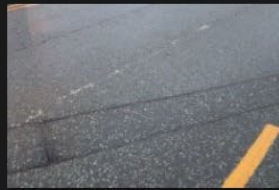
4A-4B - Rectory Lane - Road Surface - 18-01-2026 (39)
