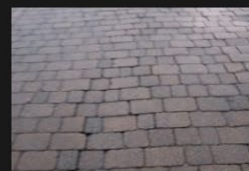
4A-4B – Rectory Lane – Road Surface - 18-01-2026 (17)
