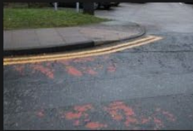
4A-4B - Rectory Lane - Road Surface - 18-01-2026 (105)
