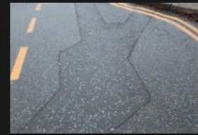
4A-4B - Rectory Lane - Road Surface - 18-01-2026 (41)
