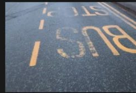
4A-4B - Rectory Lane - Road Surface - 18-01-2026 (34)
