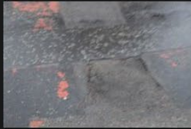
4A-4B - Rectory Lane - Road Surface - 18-01-2026 (99)
