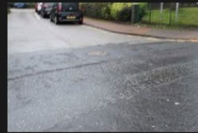
4A-4B - Rectory Lane - Road Surface - 18-01-2026 (107)
