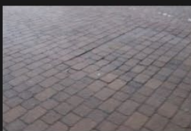
4A-4B – Rectory Lane – Road Surface - 18-01-2026 (14)
