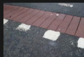
4A-4B - Rectory Lane - Road Surface - 18-01-2026 (70)
