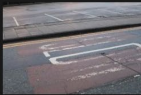
4A-4B - Rectory Lane - Road Surface - 18-01-2026 (44)
