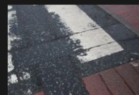
4A-4B - Rectory Lane - Road Surface - 18-01-2026 (65)
