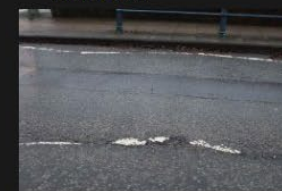
4A-4B - Rectory Lane - Road Surface - 18-01-2026 (60)
