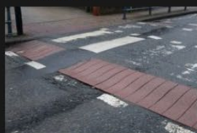
4A-4B - Rectory Lane - Road Surface - 18-01-2026 (62)
