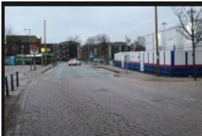
4A-4B – Rectory Lane – Road Surface - 18-01-2026 (1)
