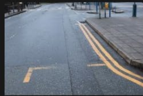
4A-4B - Rectory Lane - Road Surface - 18-01-2026 (43)
