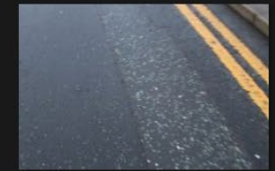
4A-4B - Rectory Lane - Road Surface - 18-01-2026 (48)
