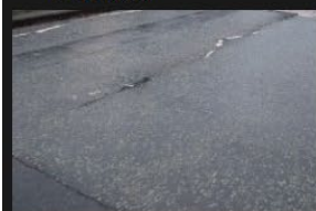
4A-4B - Rectory Lane - Road Surface - 18-01-2026 (55)
