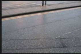
4A-4B - Rectory Lane - Road Surface - 18-01-2026 (38)
