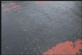
4A-4B - Rectory Lane - Road Surface - 18-01-2026 (110)
