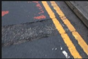
4A-4B - Rectory Lane - Road Surface - 18-01-2026 (103)
