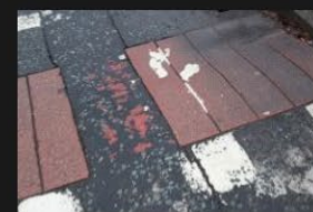
4A-4B - Rectory Lane - Road Surface - 18-01-2026 (71)
