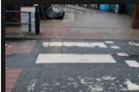
4A-4B - Rectory Lane - Road Surface - 18-01-2026 (67)
