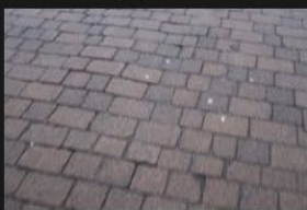
4A-4B – Rectory Lane – Road Surface - 18-01-2026 (20)
