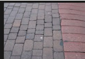
4A-4B – Rectory Lane – Road Surface - 18-01-2026 (5)
