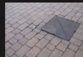
4A-4B – Rectory Lane – Road Surface - 18-01-2026 (18)
