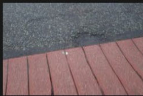
4A-4B - Rectory Lane - Road Surface - 18-01-2026 (26)
