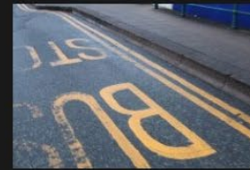
4A-4B - Rectory Lane - Road Surface - 18-01-2026 (35)
