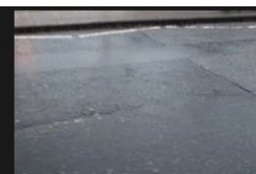
4A-4B - Rectory Lane - Road Surface - 18-01-2026 (53)
