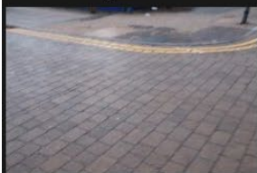
4A-4B – Rectory Lane – Road Surface - 18-01-2026 (19)
