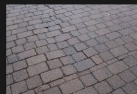
4A-4B – Rectory Lane – Road Surface - 18-01-2026 (11)
