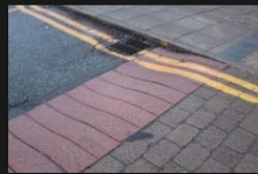
4A-4B - Rectory Lane - Road Surface - 18-01-2026 (25)
