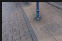
3A-3B – Rectory Lane – Kerbs and Footpath - 18-01-2026 (94)
