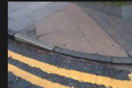
3A-3B – Rectory Lane – Kerbs and Footpath - 18-01-2026 (5)
