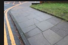
3A-3B – Rectory Lane – Kerbs and Footpath - 18-01-2026 (11)
