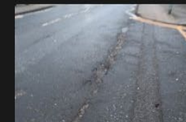
3A-3B – Rectory Lane – Kerbs and Footpath - 18-01-2026 (18)
