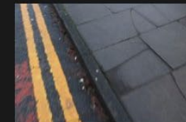
3A-3B – Rectory Lane – Kerbs and Footpath - 18-01-2026 (12)
