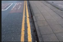
3A-3B – Rectory Lane – Kerbs and Footpath - 18-01-2026 (69)
