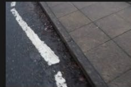
3A-3B – Rectory Lane – Kerbs and Footpath - 18-01-2026 (65)
