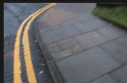
3A-3B – Rectory Lane – Kerbs and Footpath - 18-01-2026 (13)
