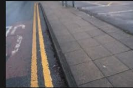
3A-3B – Rectory Lane – Kerbs and Footpath - 18-01-2026 (71)
