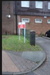
3A-3B – Rectory Lane – Kerbs and Footpath - 18-01-2026 (3)
