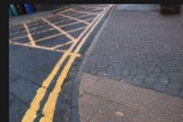
3A-3B – Rectory Lane – Kerbs and Footpath - 18-01-2026 (16)
