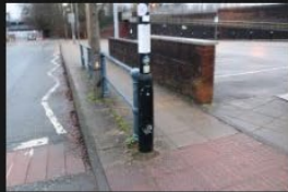
3A-3B – Rectory Lane – Kerbs and Footpath - 18-01-2026 (50)
