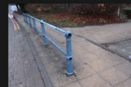
3A-3B – Rectory Lane – Kerbs and Footpath - 18-01-2026 (96)
