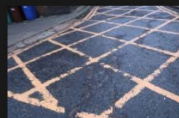
3A-3B – Rectory Lane – Kerbs and Footpath - 18-01-2026 (21)
