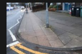
3A-3B – Rectory Lane – Kerbs and Footpath - 18-01-2026 (24)
