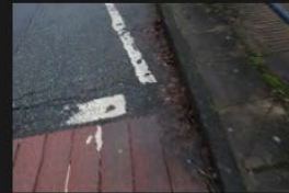
3A-3B – Rectory Lane – Kerbs and Footpath - 18-01-2026 (53)
