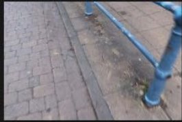
3A-3B – Rectory Lane – Kerbs and Footpath - 18-01-2026 (97)
