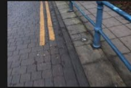
3A-3B – Rectory Lane – Kerbs and Footpath - 18-01-2026 (101)
