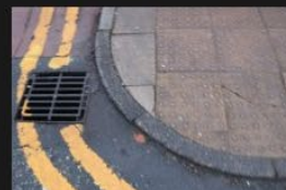
3A-3B – Rectory Lane – Kerbs and Footpath - 18-01-2026 (89)
