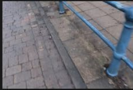
3A-3B – Rectory Lane – Kerbs and Footpath - 18-01-2026 (98)
