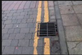
3A-3B – Rectory Lane – Kerbs and Footpath - 18-01-2026 (105)
