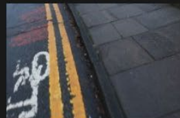
3A-3B – Rectory Lane – Kerbs and Footpath - 18-01-2026 (8)
