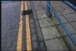
3A-3B – Rectory Lane – Kerbs and Footpath - 18-01-2026 (104)
