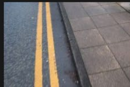
3A-3B – Rectory Lane – Kerbs and Footpath - 18-01-2026 (76)
