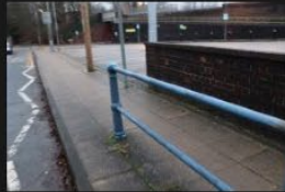
3A-3B – Rectory Lane – Kerbs and Footpath - 18-01-2026 (57)
