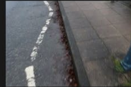
3A-3B – Rectory Lane – Kerbs and Footpath - 18-01-2026 (59)
