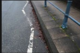
3A-3B – Rectory Lane – Kerbs and Footpath - 18-01-2026 (56)
