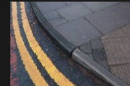
3A-3B – Rectory Lane – Kerbs and Footpath - 18-01-2026 (6)
