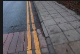
3A-3B – Rectory Lane – Kerbs and Footpath - 18-01-2026 (106)
