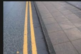
3A-3B – Rectory Lane – Kerbs and Footpath - 18-01-2026 (77)
