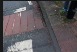
3A-3B – Rectory Lane – Kerbs and Footpath - 18-01-2026 (52)
