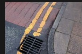
3A-3B – Rectory Lane – Kerbs and Footpath - 18-01-2026 (90)
