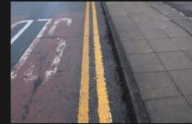
3A-3B – Rectory Lane – Kerbs and Footpath - 18-01-2026 (72)
