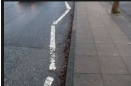
3A-3B – Rectory Lane – Kerbs and Footpath - 18-01-2026 (61)
