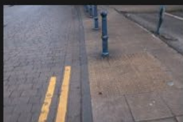
3A-3B – Rectory Lane – Kerbs and Footpath - 18-01-2026 (92)
