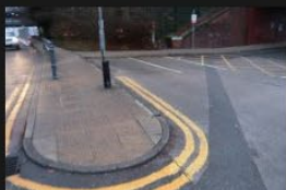
3A-3B – Rectory Lane – Kerbs and Footpath - 18-01-2026 (86)
