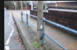
3A-3B – Rectory Lane – Kerbs and Footpath - 18-01-2026 (54)
