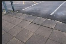
3A-3B – Rectory Lane – Kerbs and Footpath - 18-01-2026 (75)
