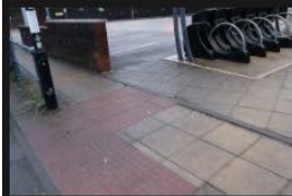
3A-3B – Rectory Lane – Kerbs and Footpath - 18-01-2026 (49)
