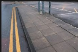
3A-3B – Rectory Lane – Kerbs and Footpath - 18-01-2026 (74)
