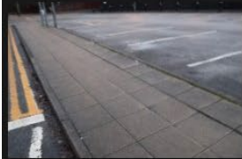
3A-3B – Rectory Lane – Kerbs and Footpath - 18-01-2026 (67)
