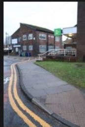
3A-3B – Rectory Lane – Kerbs and Footpath - 18-01-2026 (2)
