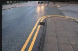
3A-3B – Rectory Lane – Kerbs and Footpath - 18-01-2026 (79)
