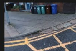
3A-3B – Rectory Lane – Kerbs and Footpath - 18-01-2026 (23)
