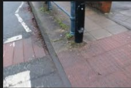
3A-3B – Rectory Lane – Kerbs and Footpath - 18-01-2026 (51)
