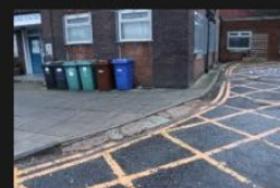
3A-3B – Rectory Lane – Kerbs and Footpath - 18-01-2026 (22)
