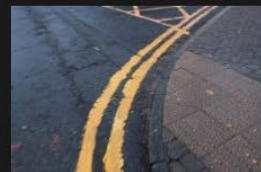
3A-3B – Rectory Lane – Kerbs and Footpath - 18-01-2026 (15)
