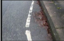
3A-3B – Rectory Lane – Kerbs and Footpath - 18-01-2026 (55)
