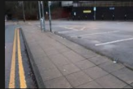
3A-3B – Rectory Lane – Kerbs and Footpath - 18-01-2026 (70)
