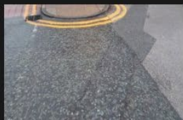
3A-3B – Rectory Lane – Kerbs and Footpath - 18-01-2026 (85)
