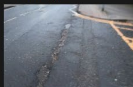
3A-3B – Rectory Lane – Kerbs and Footpath - 18-01-2026 (19)
