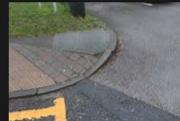
3A-3B – Rectory Lane – Kerbs and Footpath - 18-01-2026 (4)
