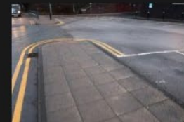
3A-3B – Rectory Lane – Kerbs and Footpath - 18-01-2026 (78)
