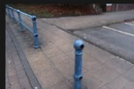
3A-3B – Rectory Lane – Kerbs and Footpath - 18-01-2026 (95)
