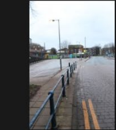
3A-3B – Rectory Lane – Kerbs and Footpath - 18-01-2026 (108)
