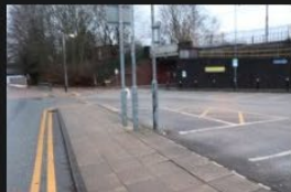
3A-3B – Rectory Lane – Kerbs and Footpath - 18-01-2026 (73)
