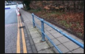
3A-3B – Rectory Lane – Kerbs and Footpath - 18-01-2026 (102)
