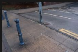
3A-3B – Rectory Lane – Kerbs and Footpath - 18-01-2026 (93)
