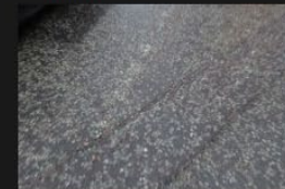
3A-3B – Rectory Lane – Kerbs and Footpath - 18-01-2026 (84)
