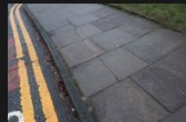
3A-3B – Rectory Lane – Kerbs and Footpath - 18-01-2026 (9)
