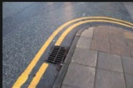
3A-3B – Rectory Lane – Kerbs and Footpath - 18-01-2026 (80)
