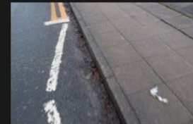
3A-3B – Rectory Lane – Kerbs and Footpath - 18-01-2026 (66)
