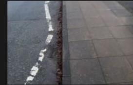
3A-3B – Rectory Lane – Kerbs and Footpath - 18-01-2026 (60)
