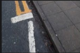
3A-3B – Rectory Lane – Kerbs and Footpath - 18-01-2026 (68)
