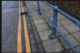
3A-3B – Rectory Lane – Kerbs and Footpath - 18-01-2026 (103)
