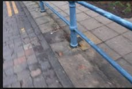
3A-3B – Rectory Lane – Kerbs and Footpath - 18-01-2026 (99)
