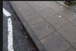
3A-3B – Rectory Lane – Kerbs and Footpath - 18-01-2026 (64)
