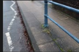
3A-3B – Rectory Lane – Kerbs and Footpath - 18-01-2026 (58)
