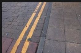
3A-3B – Rectory Lane – Kerbs and Footpath - 18-01-2026 (91)
