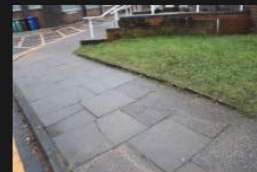
3A-3B – Rectory Lane – Kerbs and Footpath - 18-01-2026 (10)
