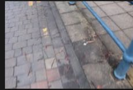
3A-3B – Rectory Lane – Kerbs and Footpath - 18-01-2026 (100)
