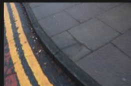
3A-3B – Rectory Lane – Kerbs and Footpath - 18-01-2026 (7)
