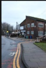
3A-3B – Rectory Lane – Kerbs and Footpath - 18-01-2026 (1)
