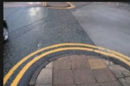
3A-3B – Rectory Lane – Kerbs and Footpath - 18-01-2026 (81)
