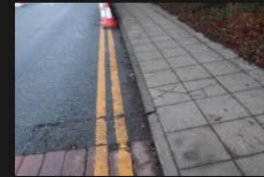
3A-3B – Rectory Lane – Kerbs and Footpath - 18-01-2026 (107)
