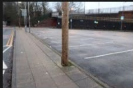
3A-3B – Rectory Lane – Kerbs and Footpath - 18-01-2026 (62)
