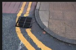
3A-3B – Rectory Lane – Kerbs and Footpath - 18-01-2026 (88)
