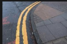
3A-3B – Rectory Lane – Kerbs and Footpath - 18-01-2026 (14)
