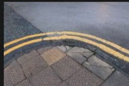
3A-3B – Rectory Lane – Kerbs and Footpath - 18-01-2026 (82)
