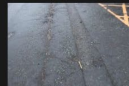
3A-3B – Rectory Lane – Kerbs and Footpath - 18-01-2026 (17)
